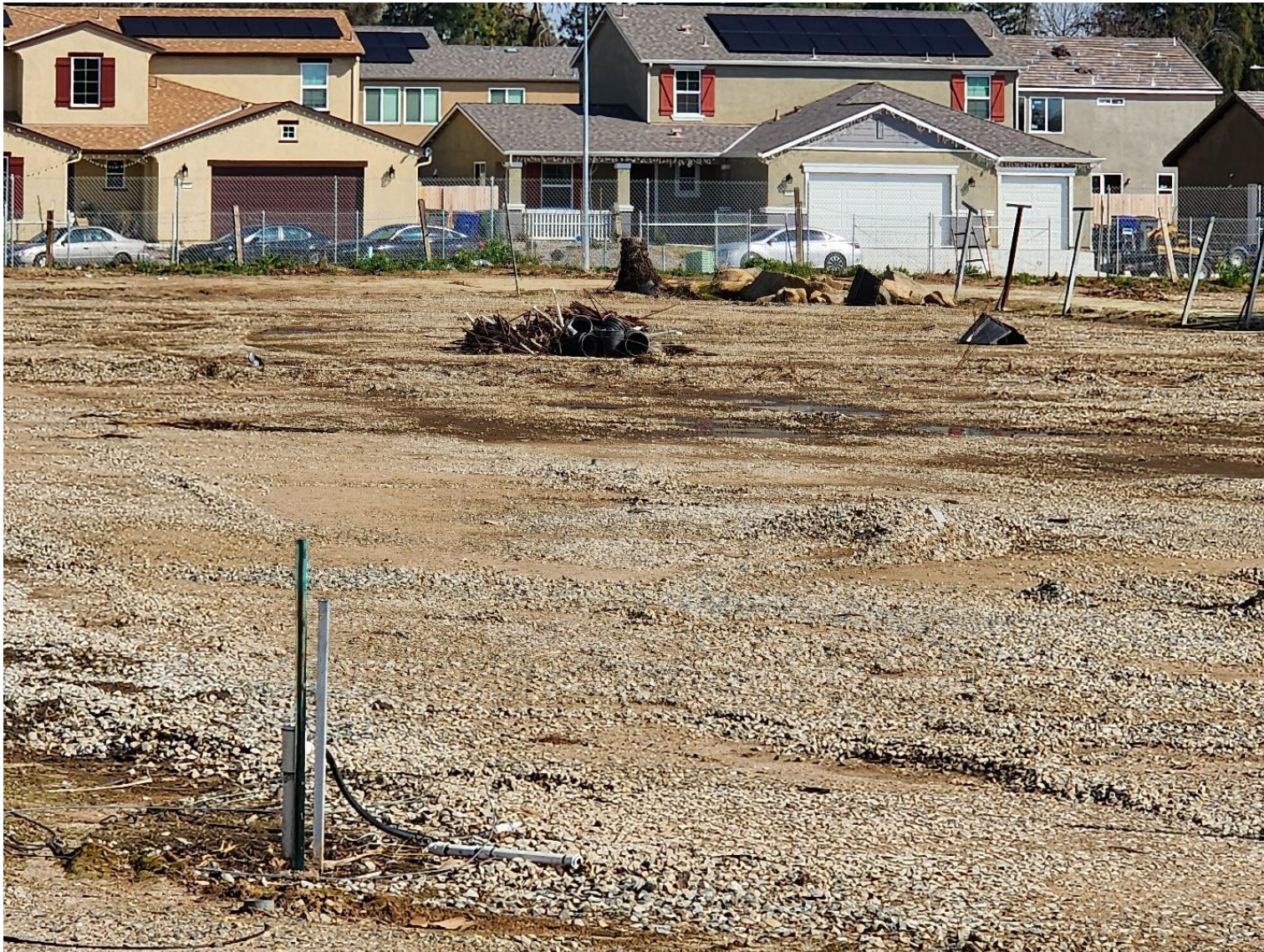
Figure 4-2 Middle of the Project Site Looking East Source: Photo by Precision Civil Engineer, Inc., on March 4, 2023
