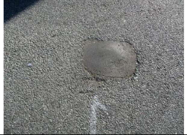
Former monitoring well BC-4 within Old Middlefield Way.
