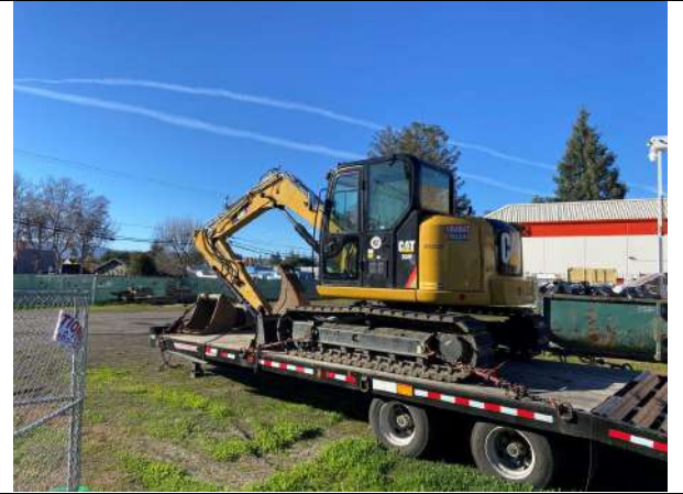
Backhoe at the northeast portion of the site.
