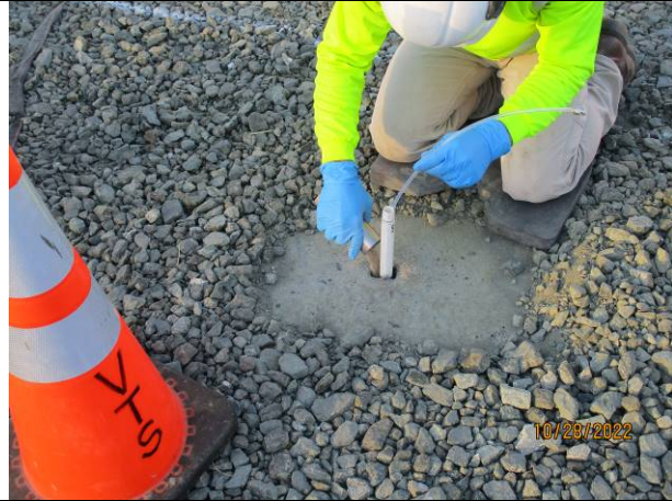
Constructing soil gas well at sample location SV1
