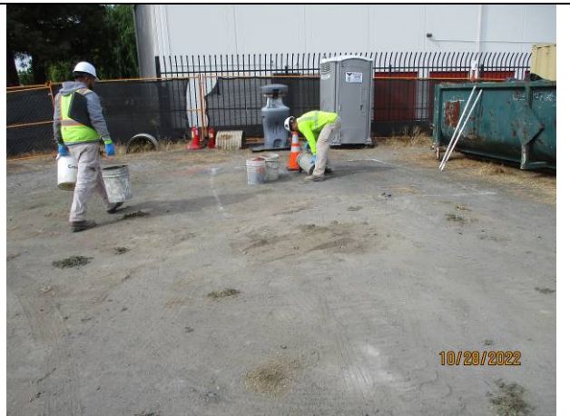
Backfilling borehole SB2
