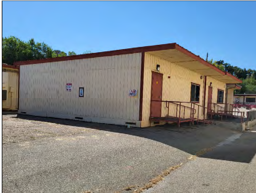
Figure 33. I-19b and I-19c Overview (view southeast; June 29, 2023)
