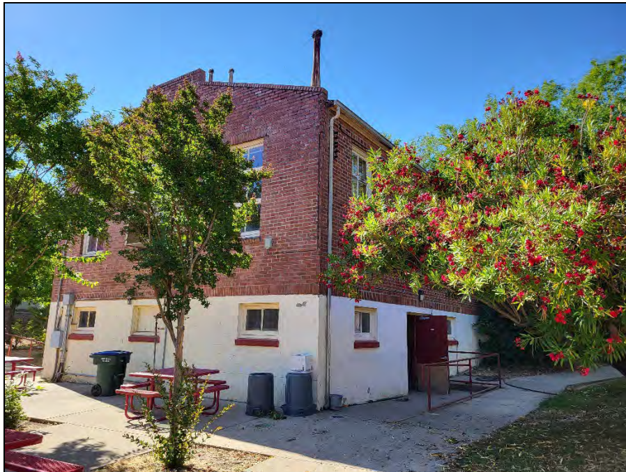
Figure 18. I-07 Overview (view southeast; June 29, 2023)
