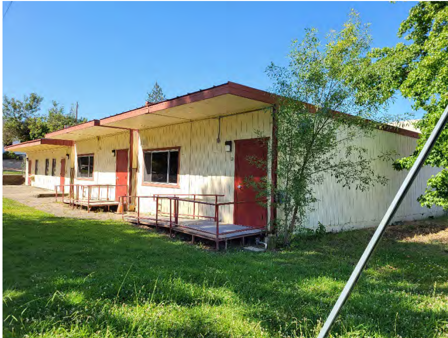
Figure 22. I-18b and I-18c Overview (view southwest; June 29, 2023)
