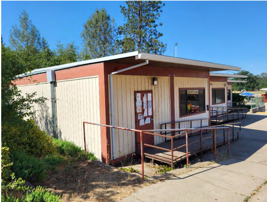
Figure 28. I-24a, I-24b, I-24c Overview (view southwest; June 29, 2023)
