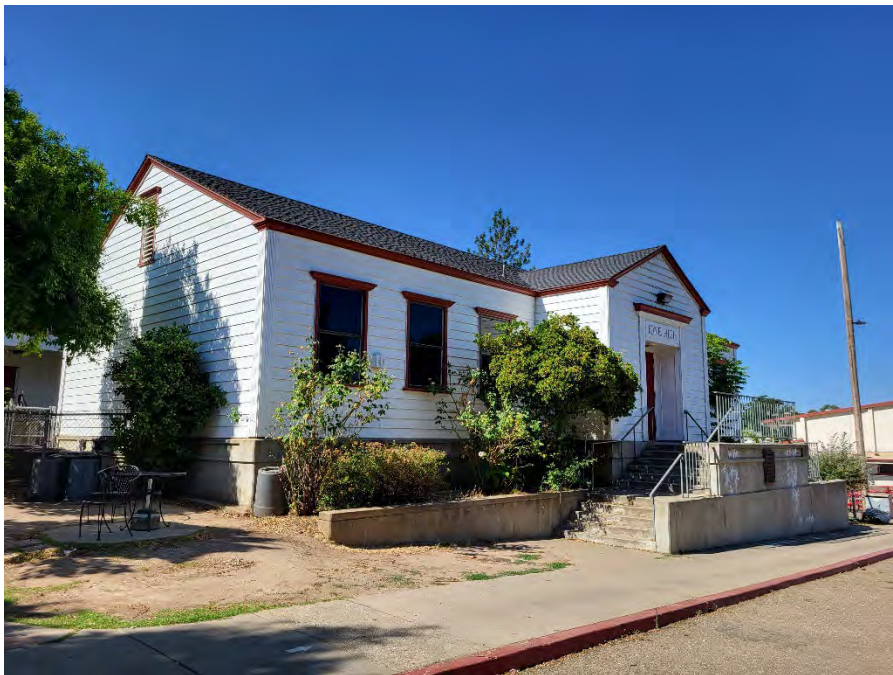
Figure 13. I-11 Overview (view southwest; June 29, 2023)
