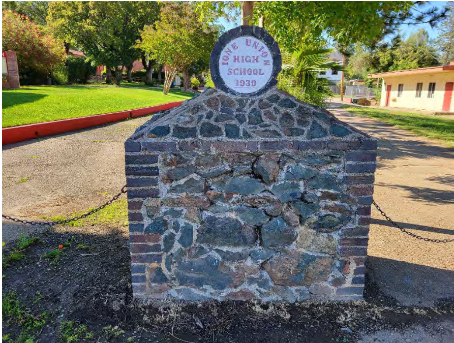
Figure 4. I-04 Overview (view south; June 29, 2023)
