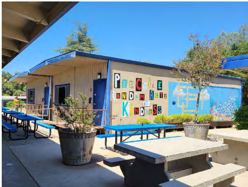
Figure 3. S-02a and S-02b Overview (view northeast; June 29, 2023)
