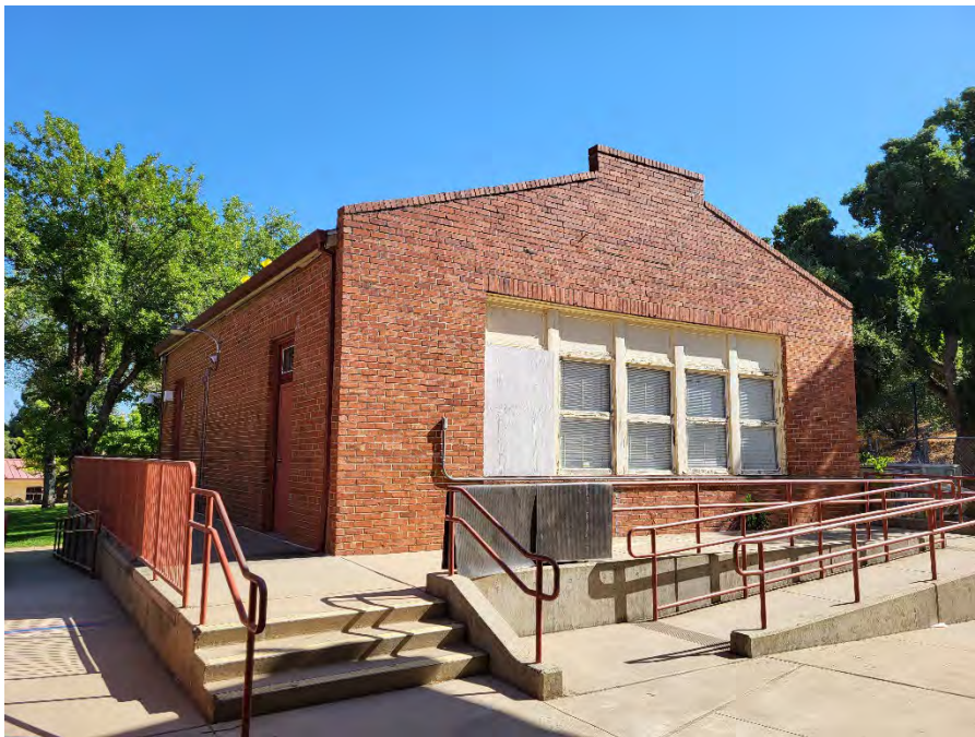
Figure 11. I-09 Overview (view north; June 29, 2023)
