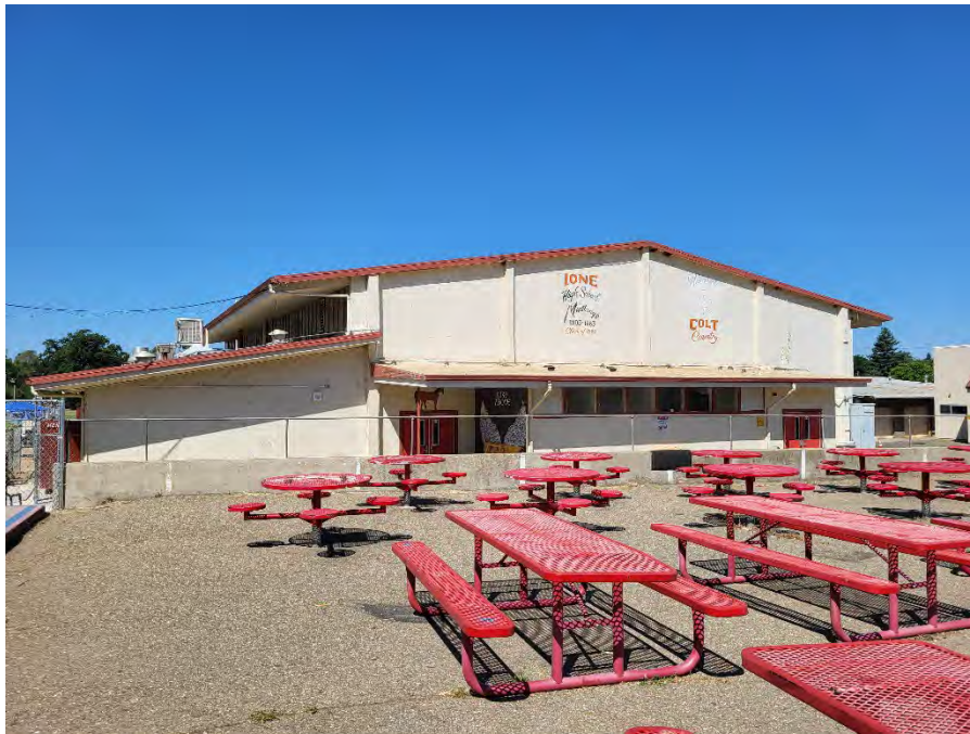
Figure 26. I-22 Overview (view west; June 29, 2023)
