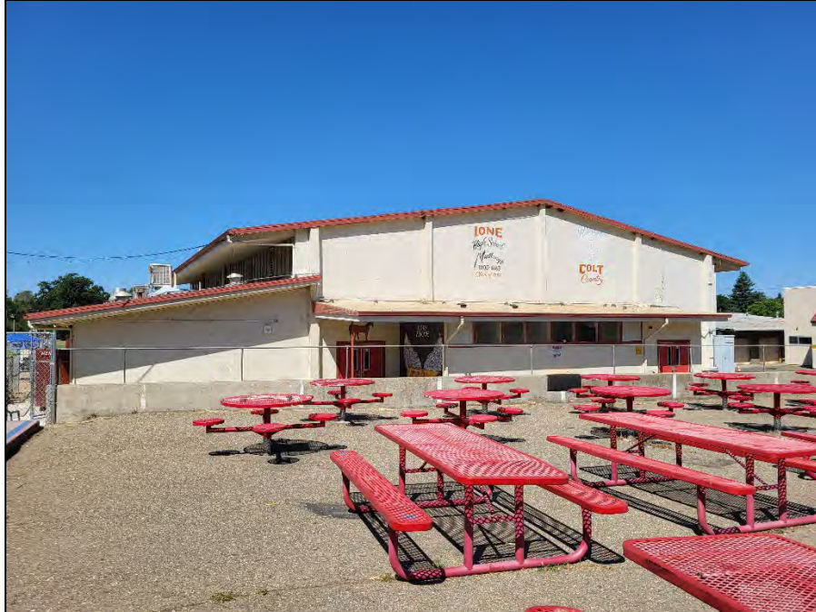
Figure 36. I-22 Overview (view west; June 29, 2023)
