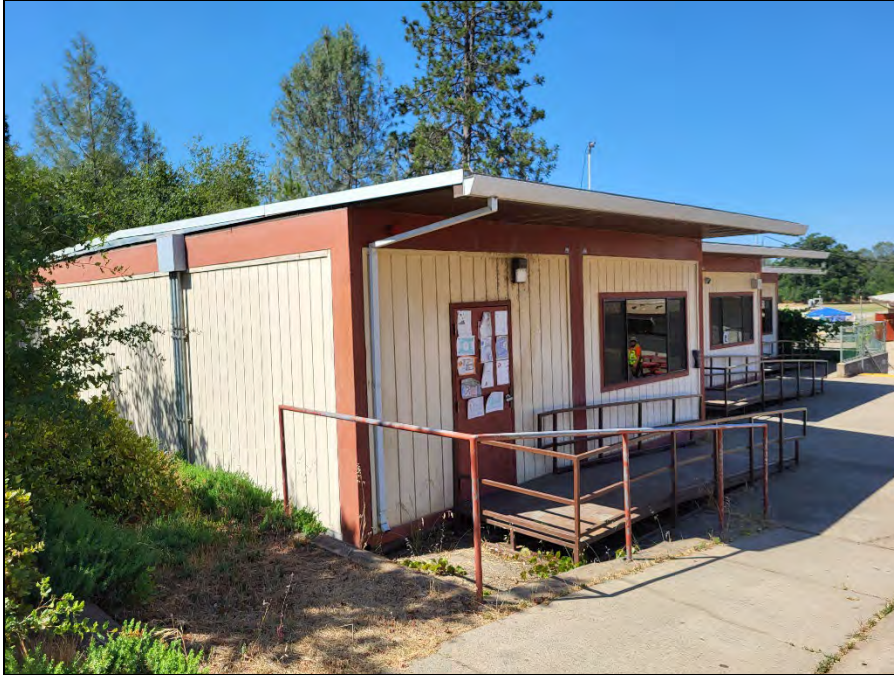
Figure 38. I-24a, I-24b, I-24c Overview (view southwest; June 29, 2023)
