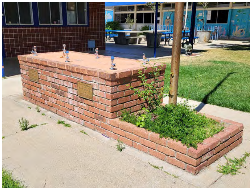
Figure 49. S-10 Overview (view northeast; June 29, 2023)
