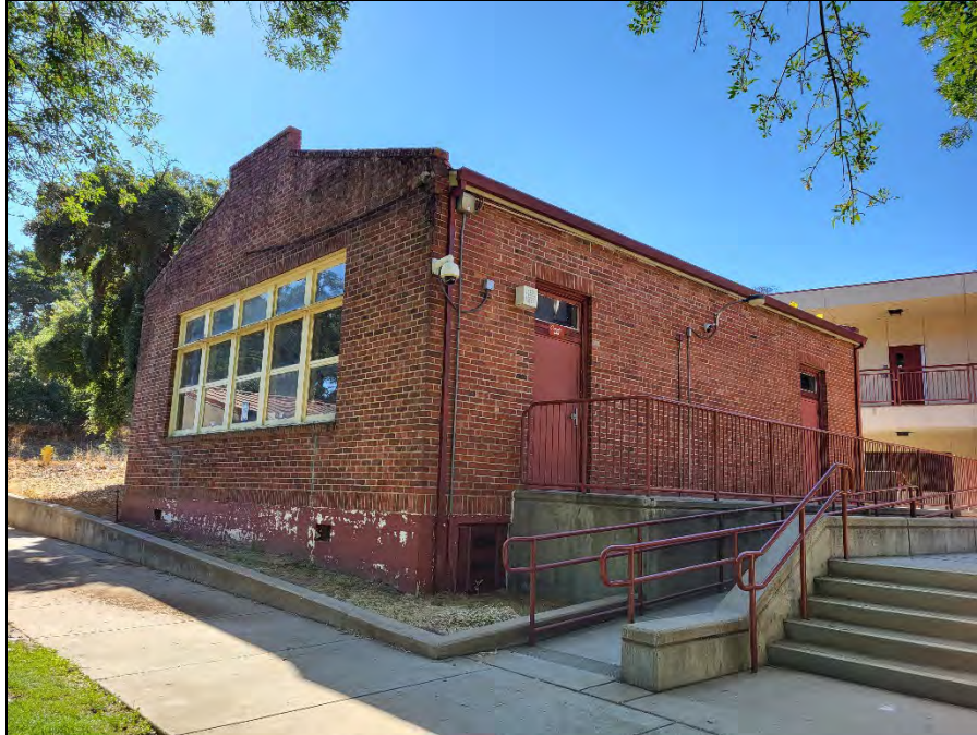
Figure 20. I-09 Overview (view southeast; June 29, 2023)
