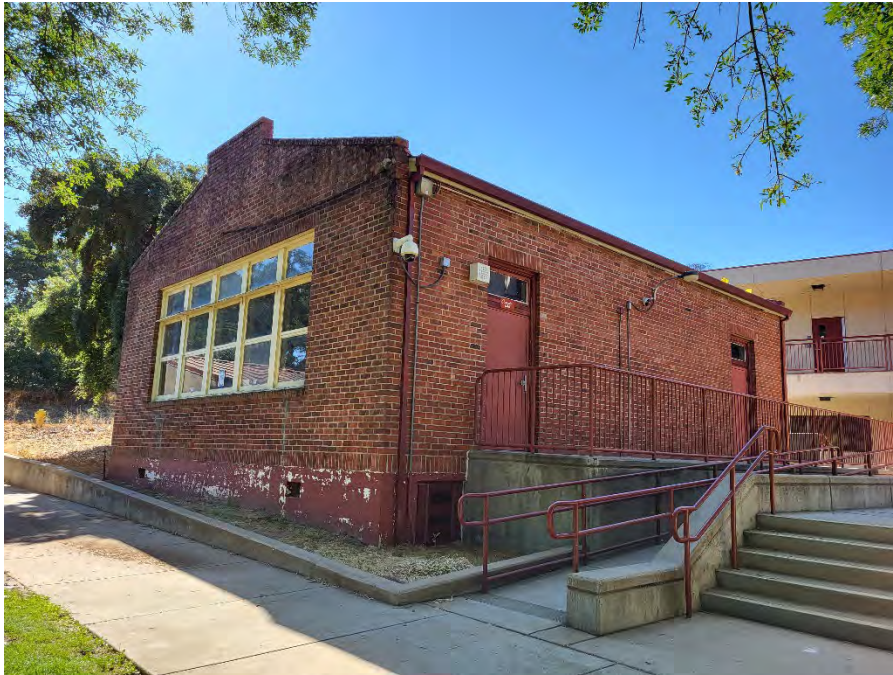
Figure 10. I-09 Overview (view southeast; June 29, 2023)
