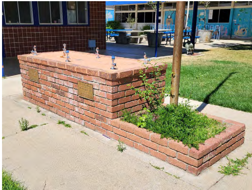
Figure 12. S-10 Overview (view northeast; June 29, 2023)
