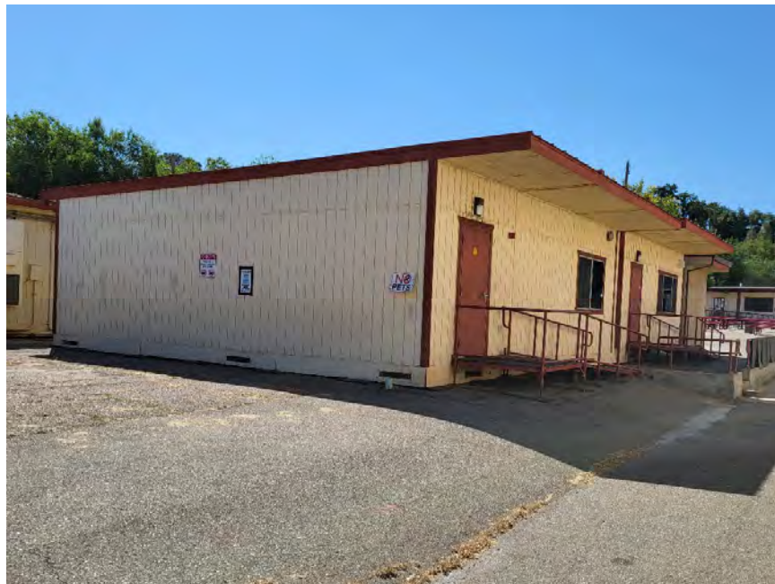
Figure 23. I-19b and I-19c Overview (view southeast; June 29, 2023)
