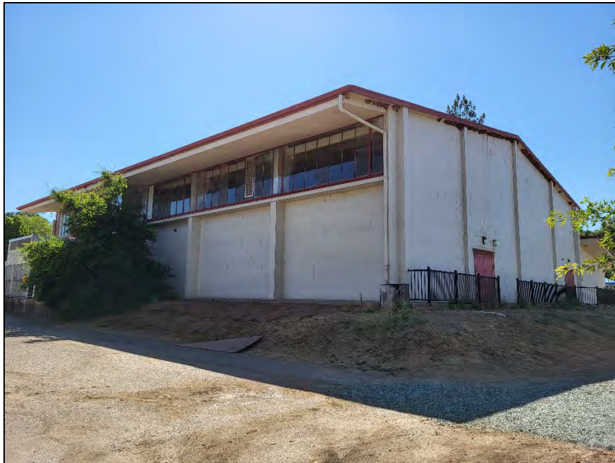
Figure 37. I-22 Overview (view east; June 29, 2023)
