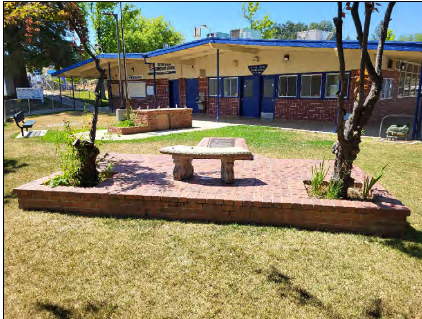
Figure 50. S-11 Overview (view northwest; June 29, 2023)
