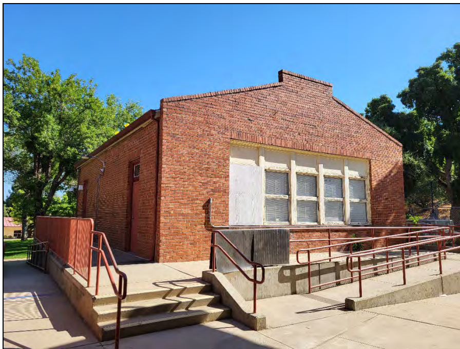
Figure 21. I-09 Overview (view north; June 29, 2023)
