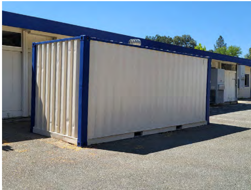
Figure 8. S-05 Overview (view northwest; June 29, 2023)
