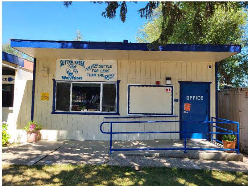
Figure 11. S-09b Overview (view east; June 29, 2023)
