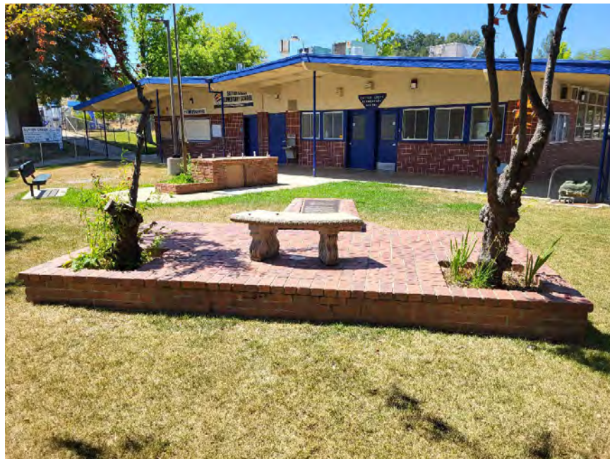
Figure 13. S-11 Overview (view northwest; June 29, 2023)
