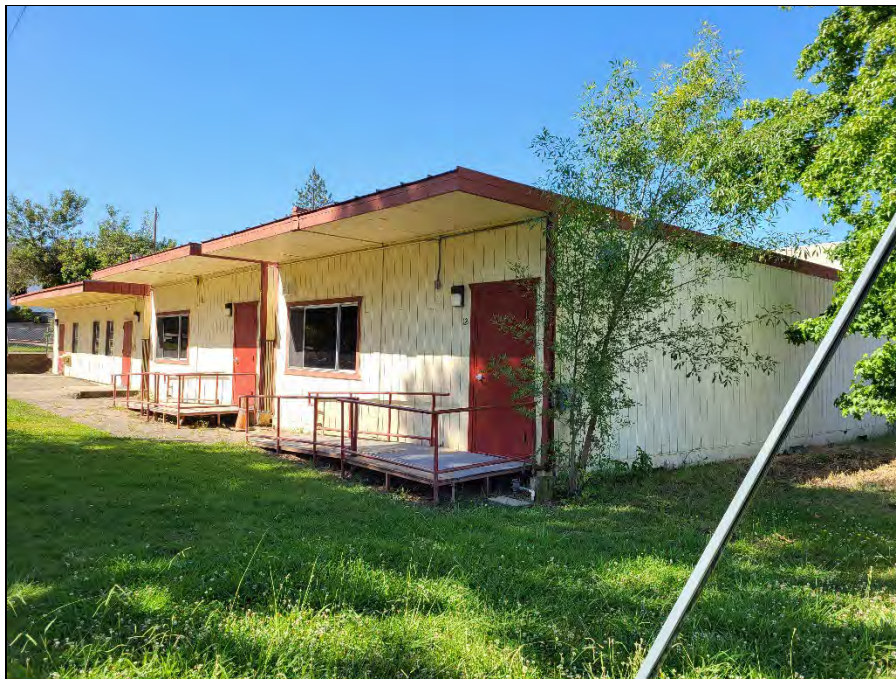
Figure 32. I-18b and I-18c Overview (view southwest; June 29, 2023)
