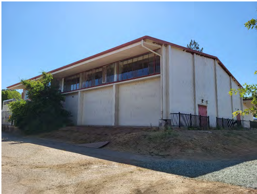
Figure 27. I-22 Description (June 29; 2023)
