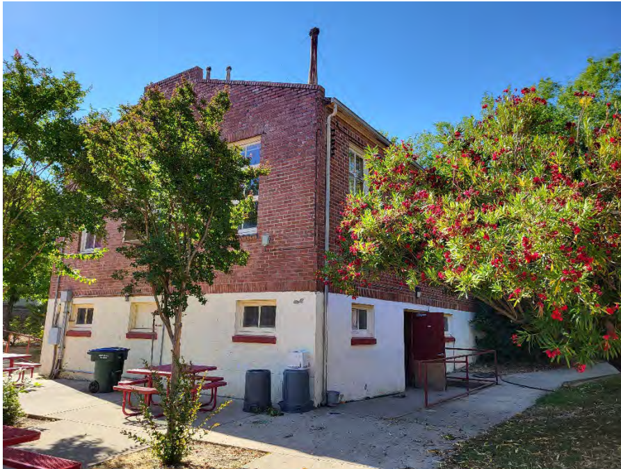
Figure 8. I-07 Overview (view southeast; June 29, 2023)
