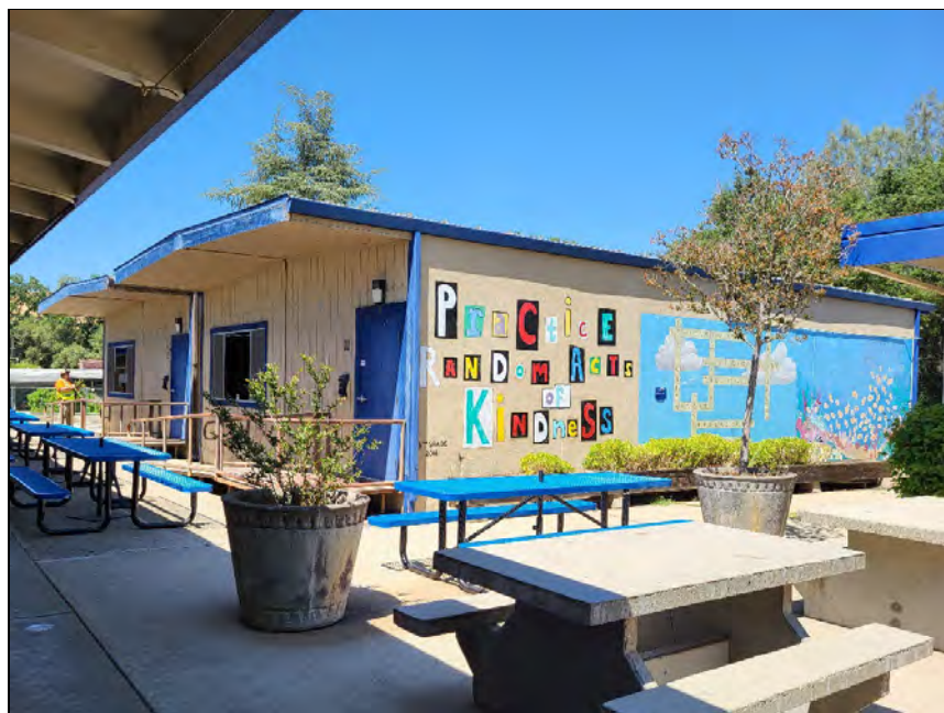
Figure 40. S-02a and S-02b Overview (view northeast; June 29, 2023)
