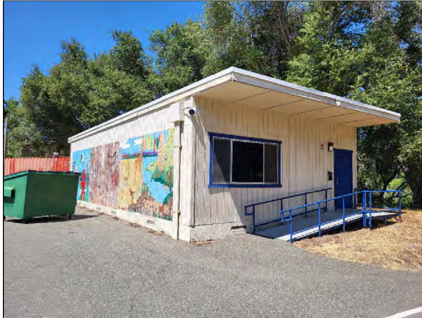
Figure 41. S-03 Overview (view northeast; June 29, 2023)
