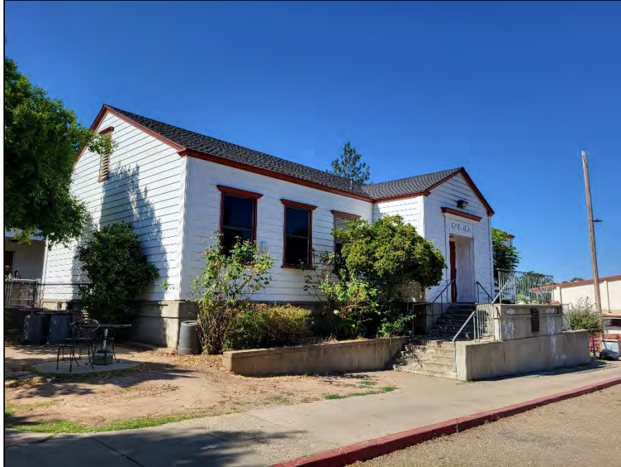
Figure 23. I-11 Overview (view southwest; June 29, 2023)
