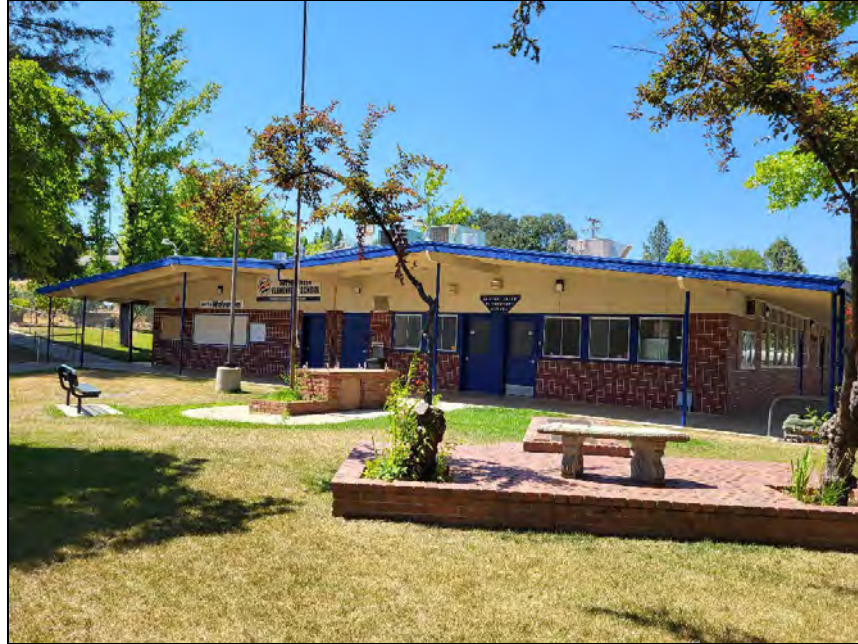
Figure 39. S-01 Overview (view northwest; June 29, 2023)
