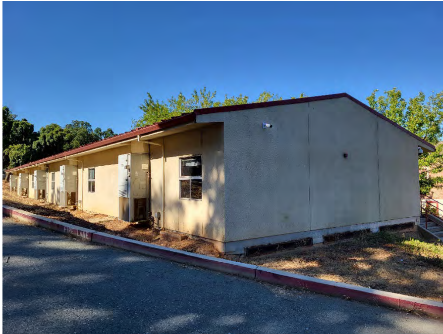
Figure 2. I-02 Overview (view southwest; June 29, 2023)
