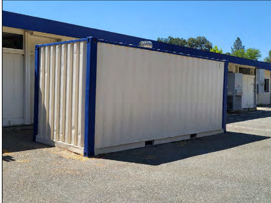
Figure 45. S-05 Overview (view northwest; June 29, 2023)
