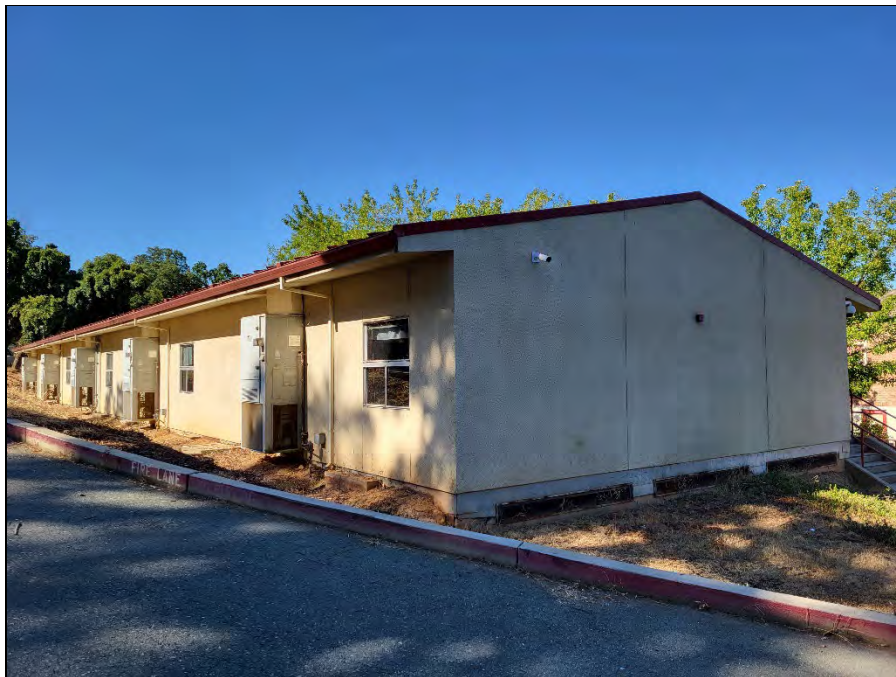
Figure 12. I-02 Overview (view southwest; June 29, 2023)
