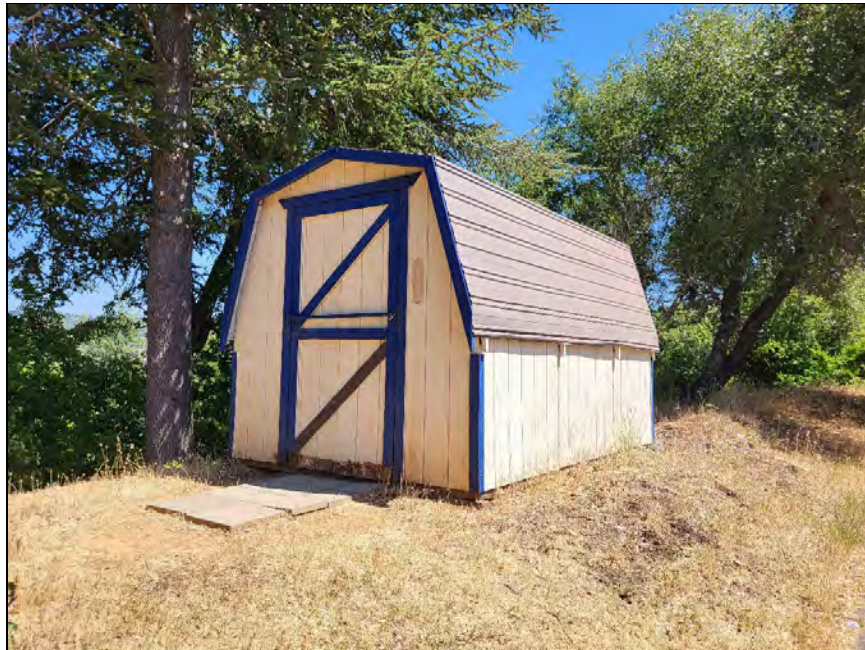
Figure 43. S-05 Overview (view southeast; June 29, 2023)
