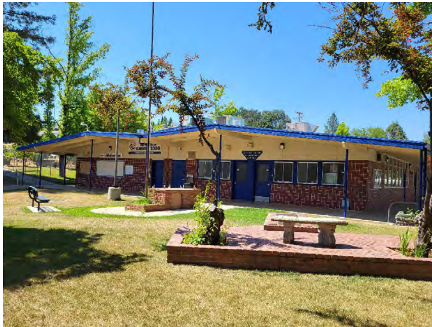
Figure 2. S-01 Overview (view northwest; June 29, 2023)
