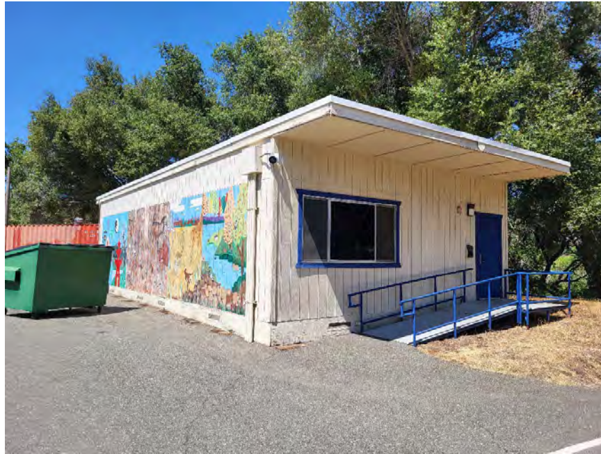
Figure 4. S-03 Overview (view northeast; June 29, 2023)
