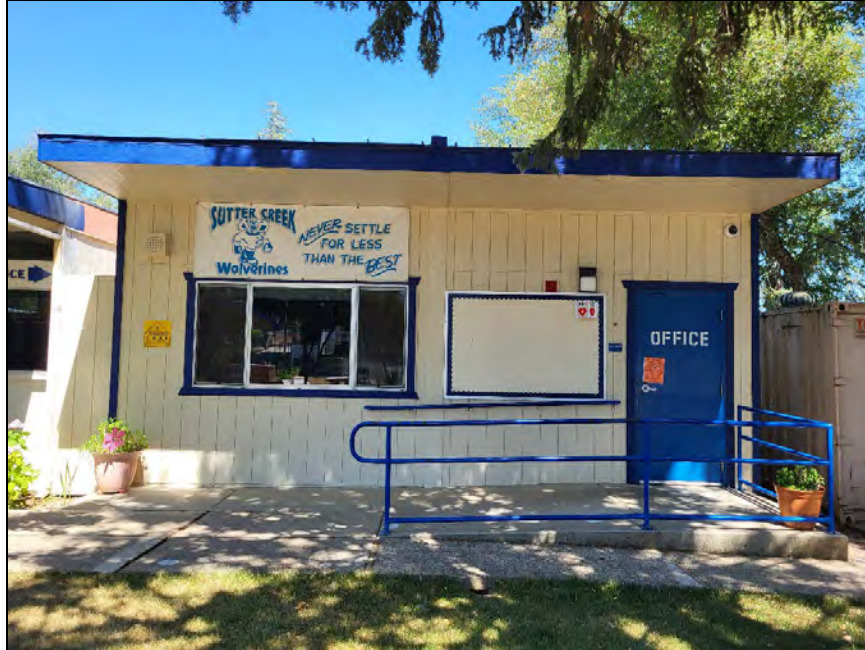
Figure 48. S-09b Overview (view east; June 29, 2023)
