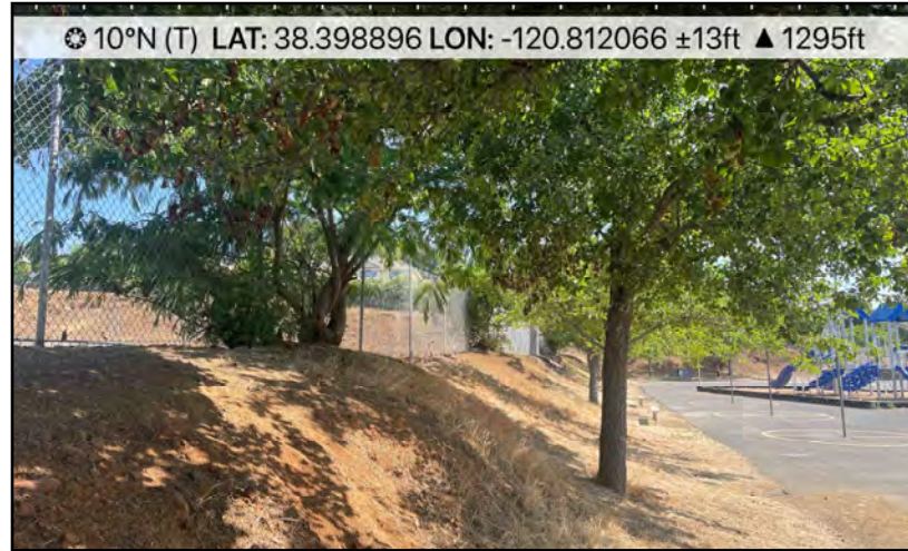
Photo 2. Representative photo of the dirt border between the playground and sports field in the BSA. Photo taken June 23, 2023, facing north.
