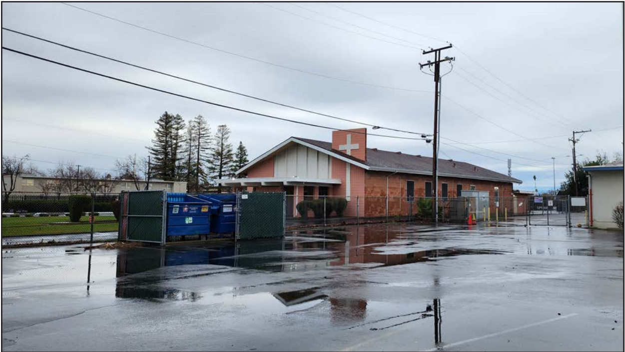
Church north of site.
