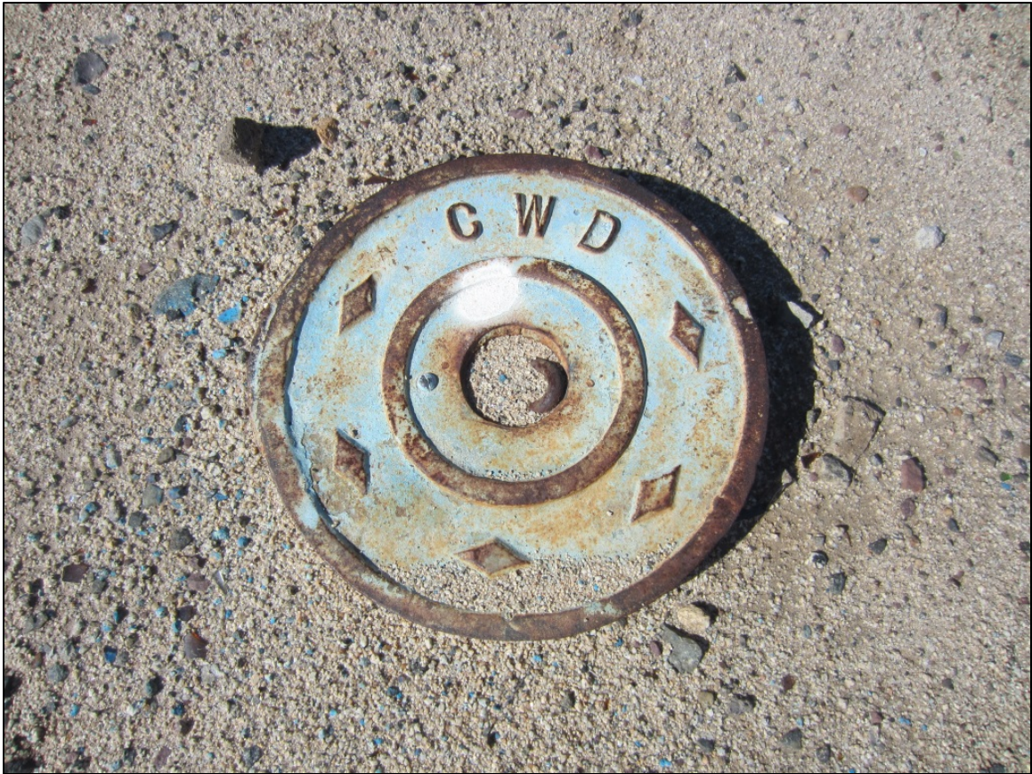
Figure 2: Detail of Hydrant Valve Cover
