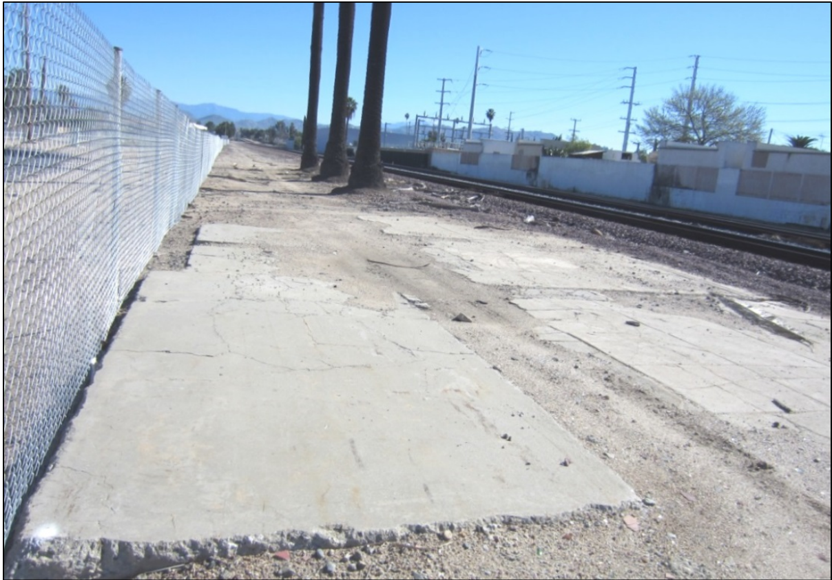
Figure 4: Concrete Foundation, facing east.
