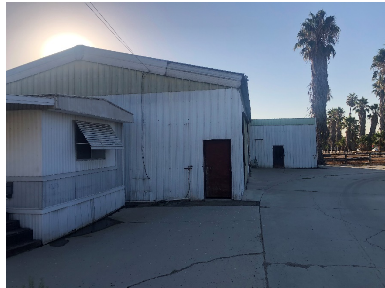
Photo 4: Sheds / Storage East of Dairy Building
