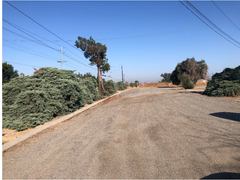
Photo 1: Dallape Dairy access road
