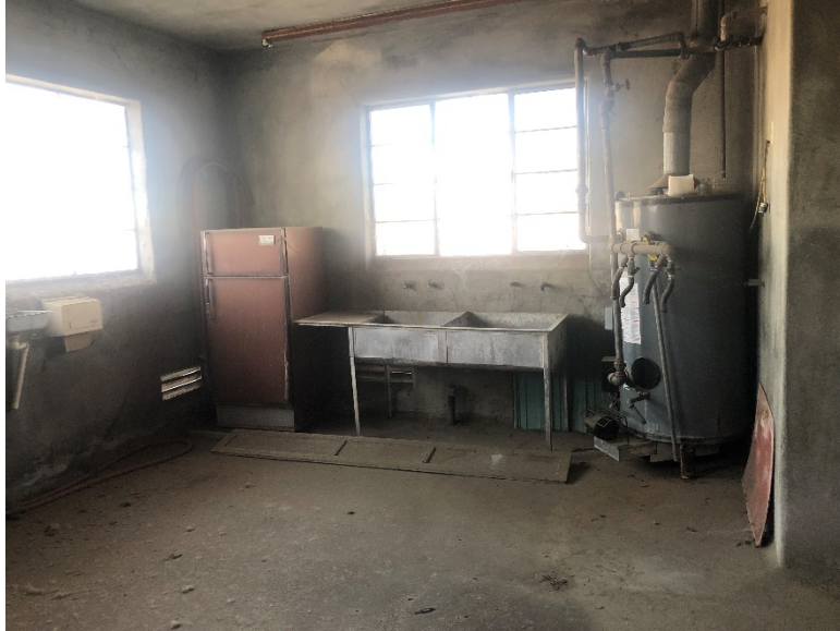
Photo 5: Dairy Building room
