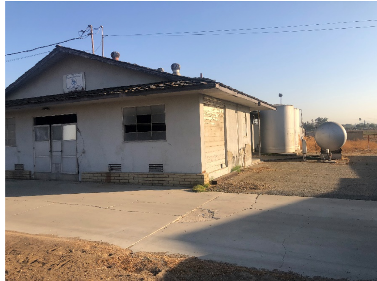
Photo 2: Dallape Dairy & water well
