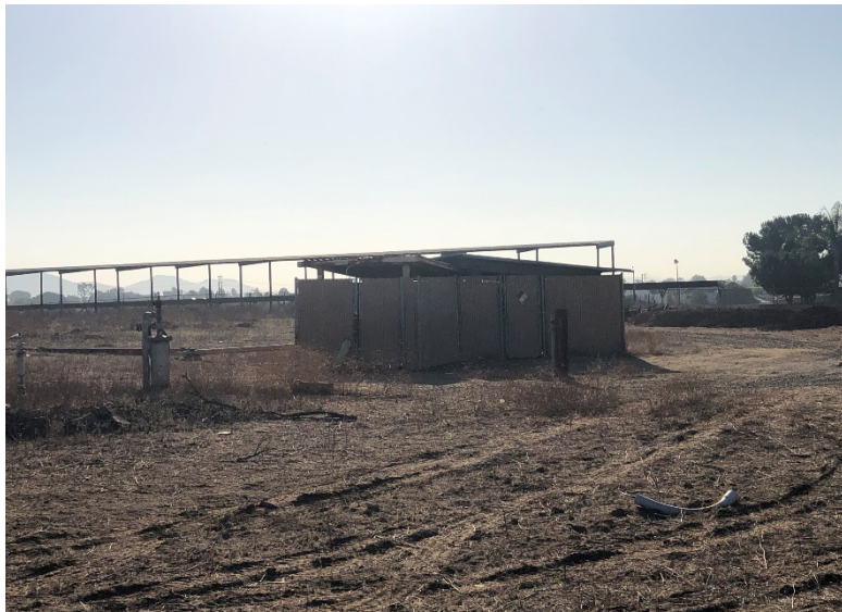
Photo 27: Well shed West end Northern parcel
