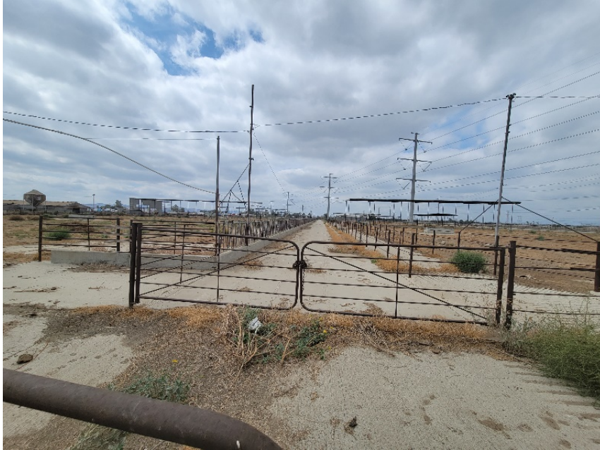
Dairy entrance SW Site; View to NE
