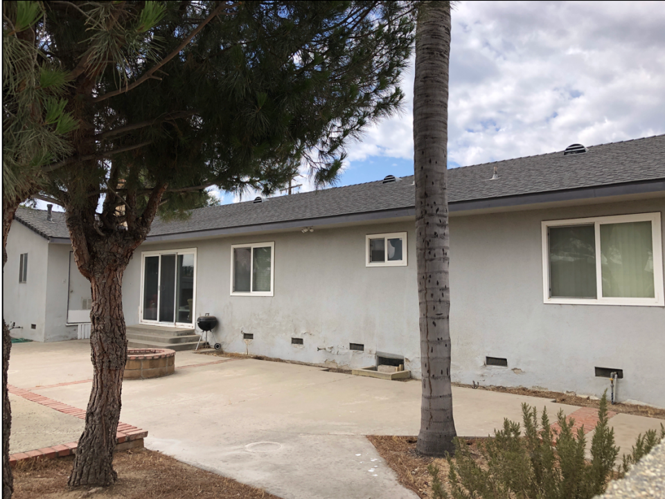
View southwest of the rear (east) elevation.
