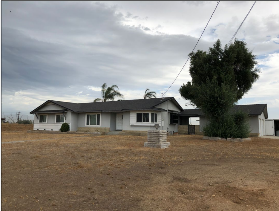
View east of the main (west) elevation.
