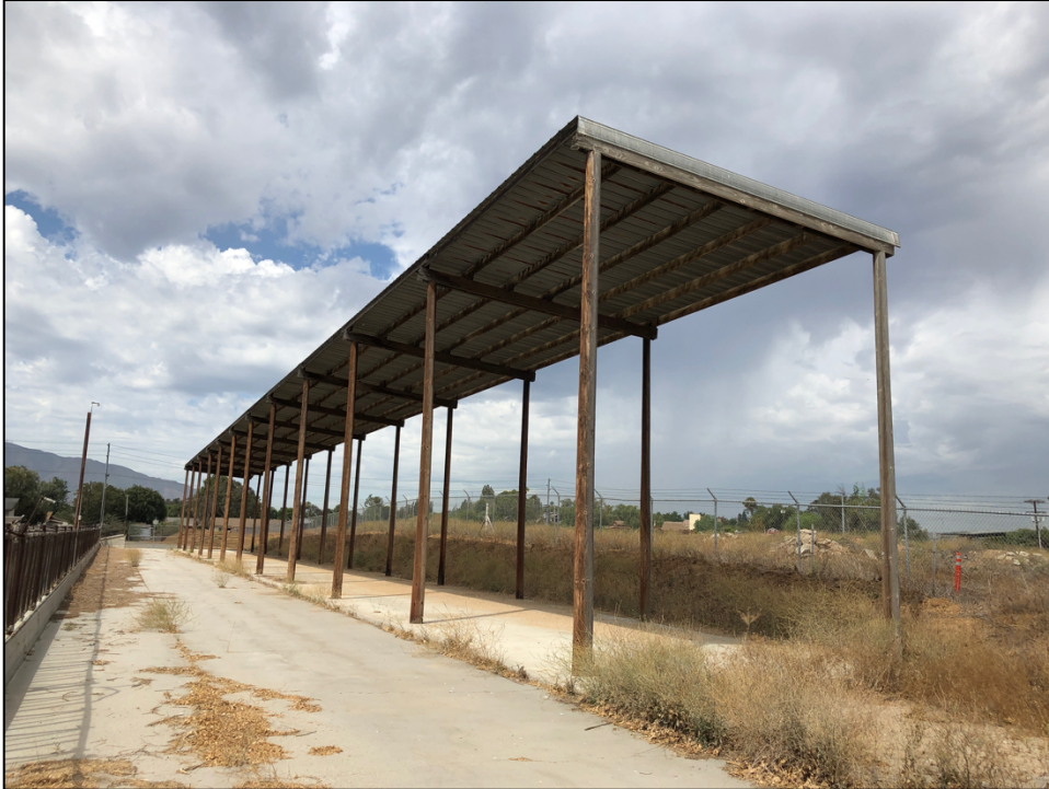
View west of pole structure with flat roof.
