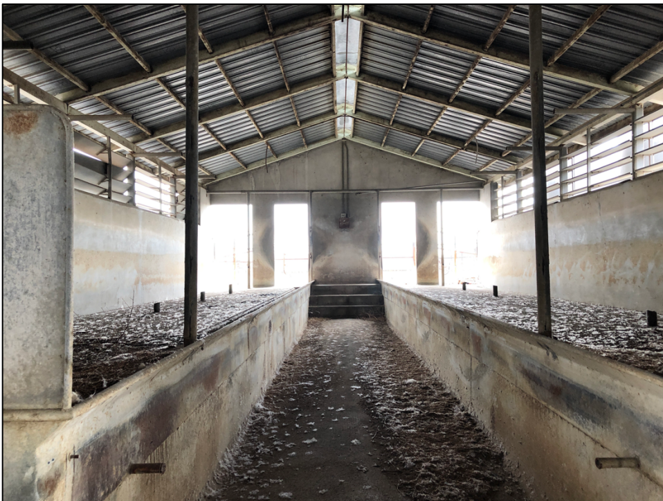
Interior view of the milk parlor's rear section. The milk parlor was constructed in the herringbone style. The herringbone style allowed milkers to more efficiently milk cows without having to kneel because the cows were at an elevated height.
