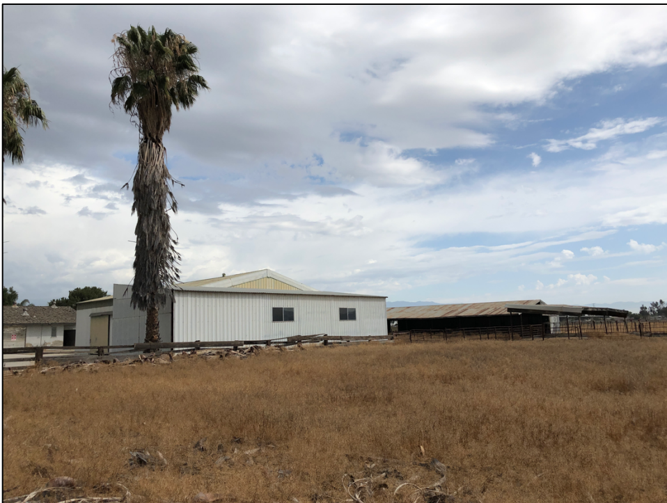
View northeast of the south elevation. A manufactured trailer is appended to the south elevation.
