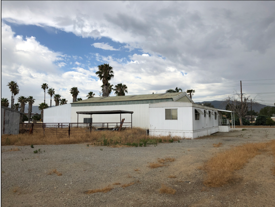
View southwest of the rear (east) elevation and partial north elevation.
