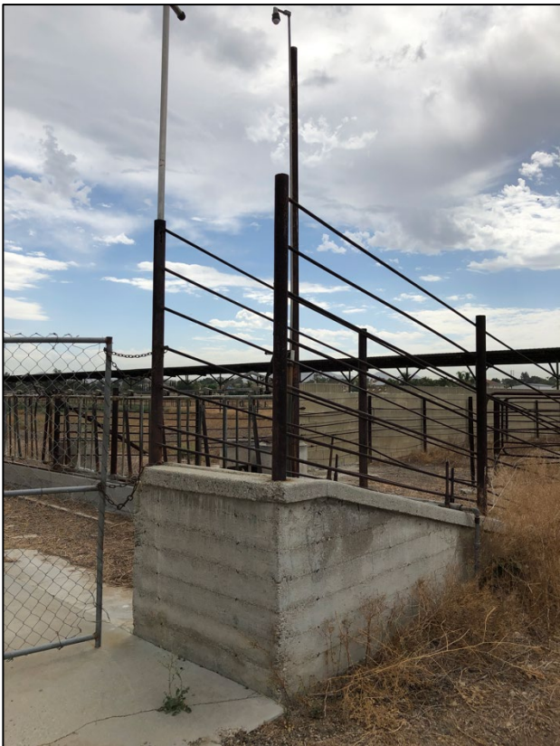
Detail view of concrete cattle loading chute located behind the main residence.
