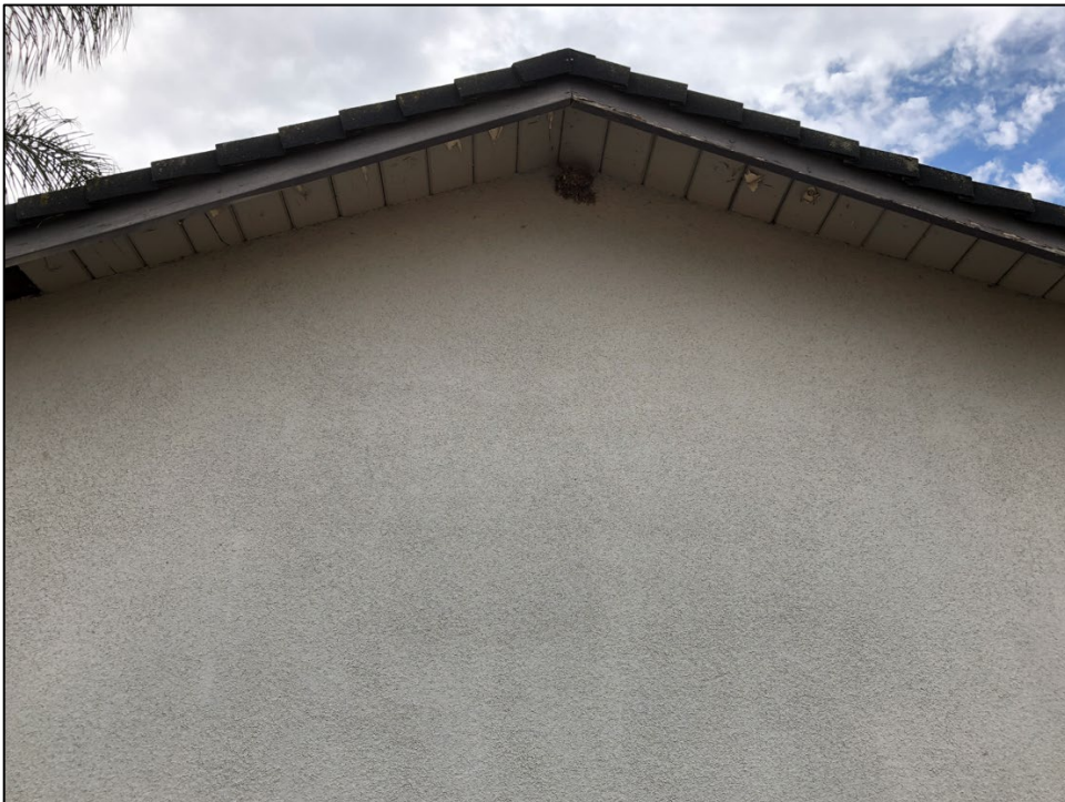
View south of the north elevation gable side.
