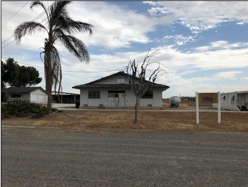
View east from driveway of the milk parlor's main (west) elevation. The milk parlor is located directly south of the main residence. Many post-1950s dairy properties have a circular driveway in front of the milk parlor to allow large semi-trucks easy access on and off the property.
