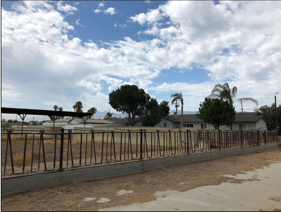
View southwest of the east elevation. Pole structure is visible in the background.
