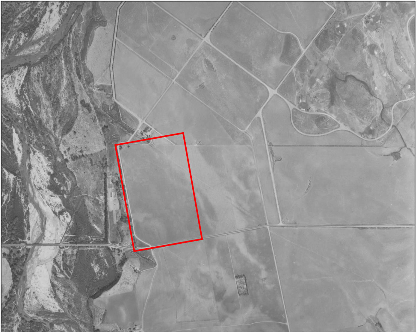
1931 aerial image of the subject property and the surrounding area. Source: Frame Finder.
