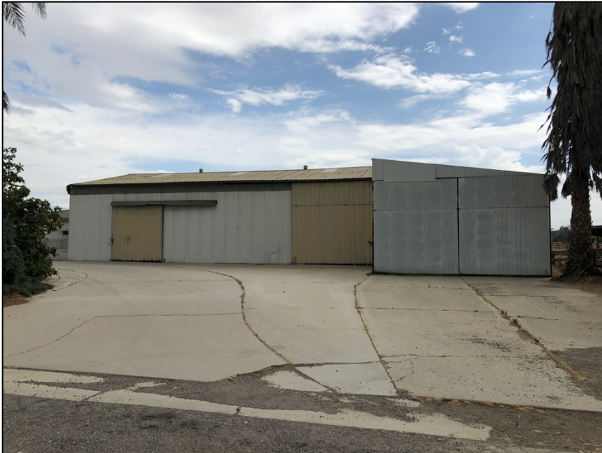
View east of the barn's main (west) elevation. The barn is located directly south of the milk parlor and features a coregulated sheet metal façade and roof.
