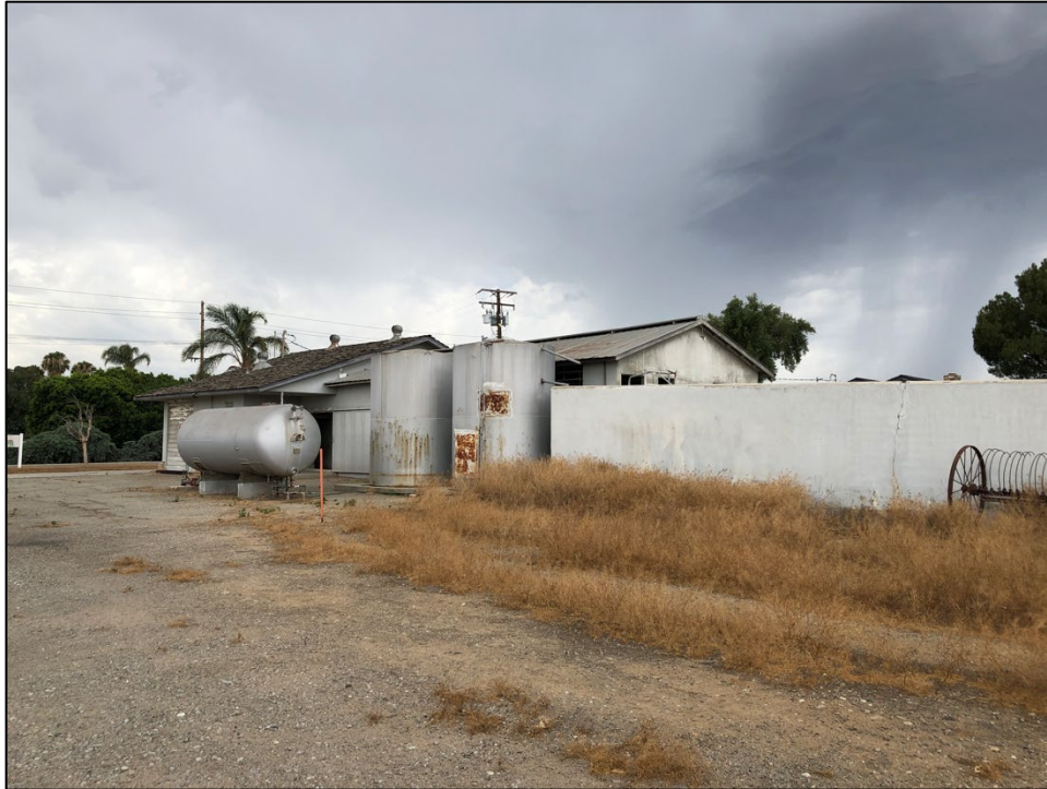
View northwest of the milk parlor's partial south and east elevations. Large silos are visible in the background.
