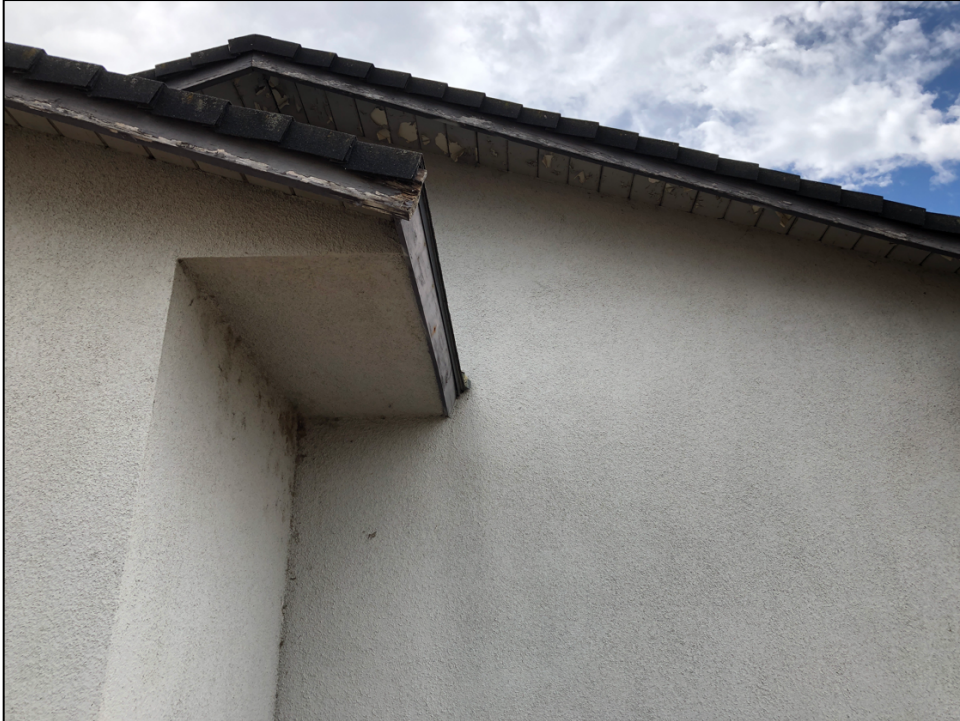
View south of the north elevation roof line.
