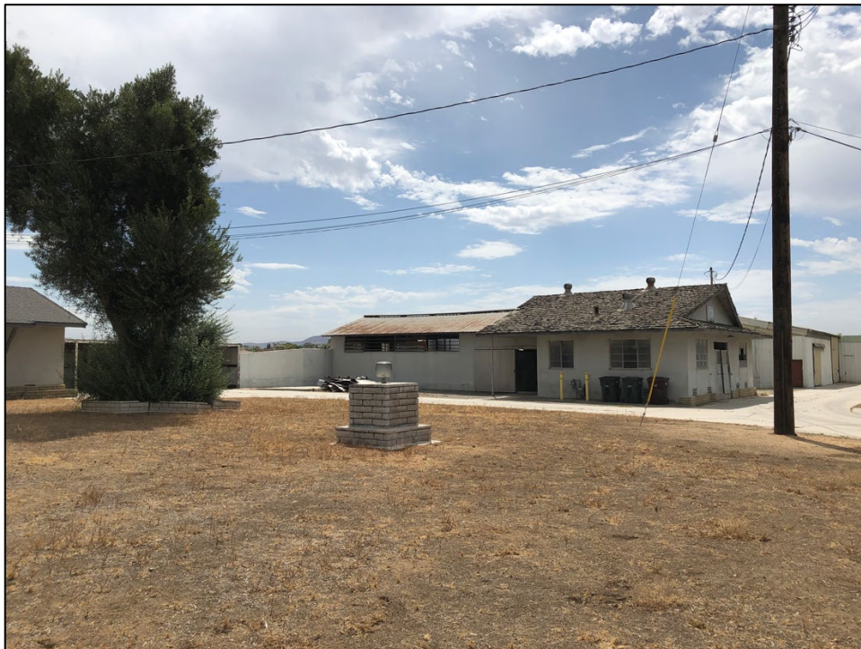
View southeast of the milk parlor's north elevation and partial west elevation.
