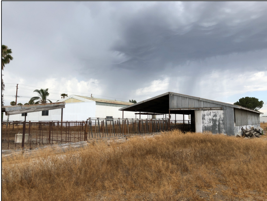
View southwest of stall structure located behind the barn and milk parlor. Corrals are visible in the background.
