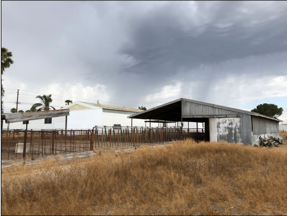
View southwest of stall structure located behind the barn and milk parlor. Corrals are visible in the background.
