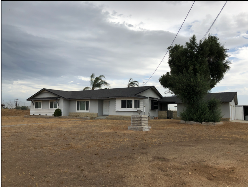
View east of the main (west) elevation.
