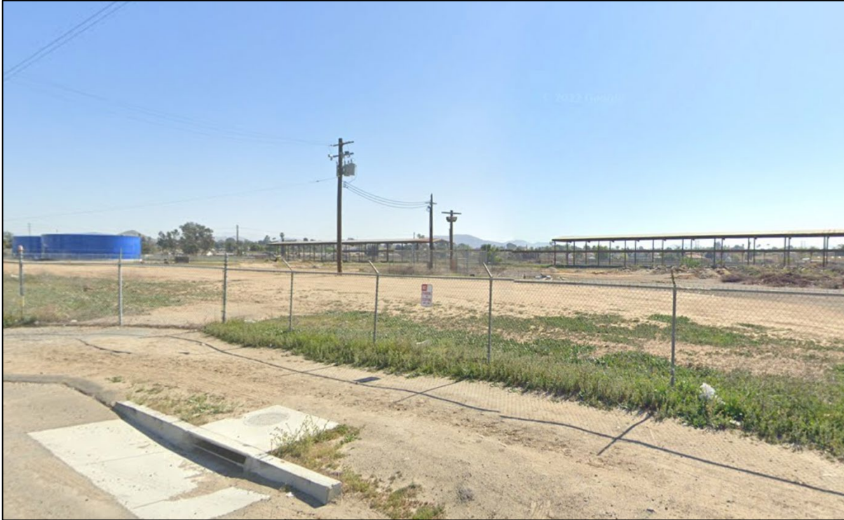
View southeast of the subject property. The wells are no longer visible on the property. The city water facility is visible in the background.
