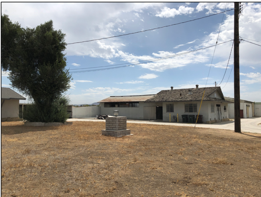
View southeast of the milk parlor's north elevation and partial west elevation
