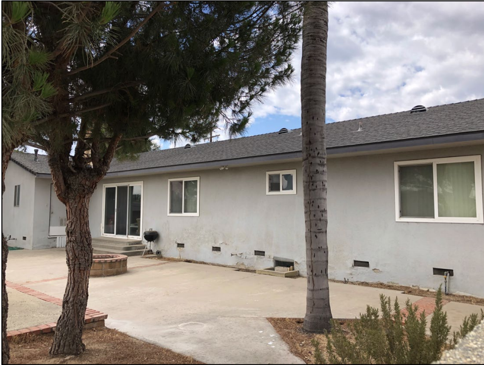
View southwest of the rear (east) elevation.
