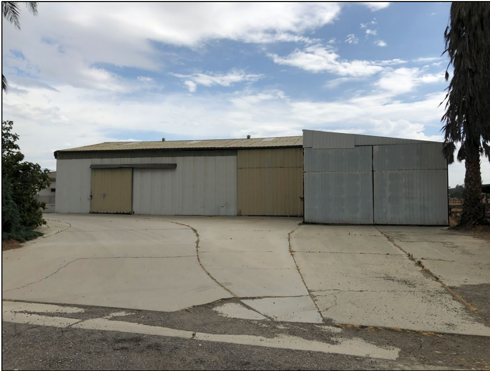
View east of the barn's main (west) elevation. The barn is located directly south of the milk parlor and features a coregulated sheet metal façade and roof.
