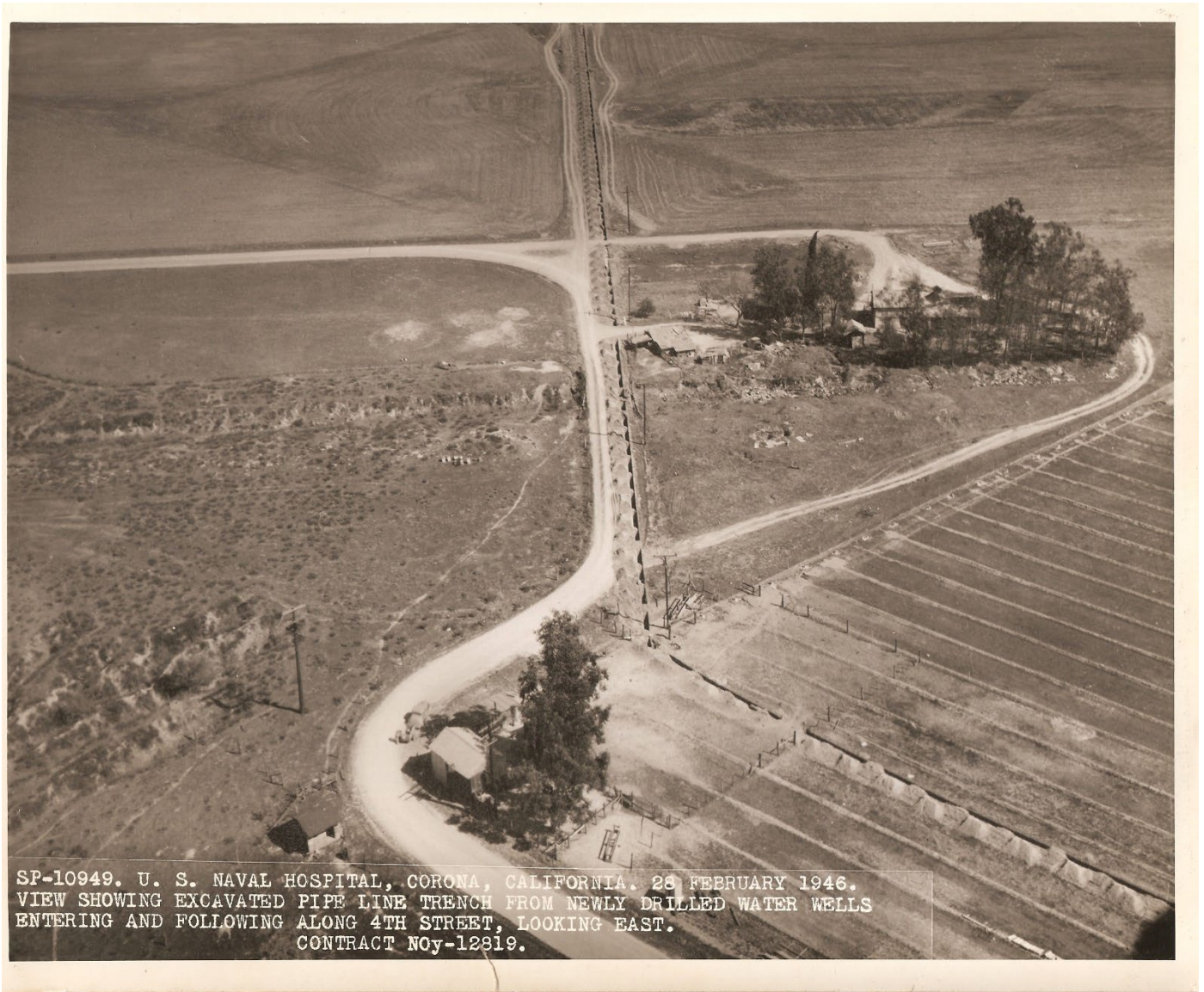
View showing excavated pipeline trench from newly drilled water wells entering and following along 4th Street, looking east. SP-10949; 2-28-1946. Source: Sea Bee Archives, courtesy Kevin Bash.
