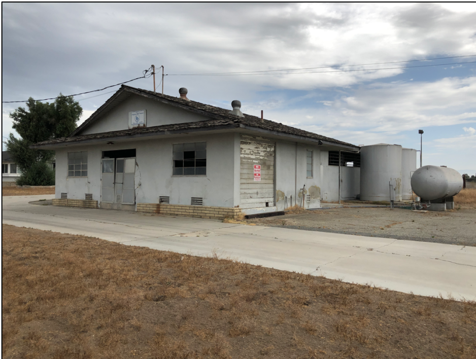
View northeast of the milk parlor's partial west and south elevations.
