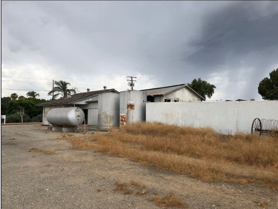
View northwest of the milk parlor's partial south and east elevations. Large silos are visible in the background.
