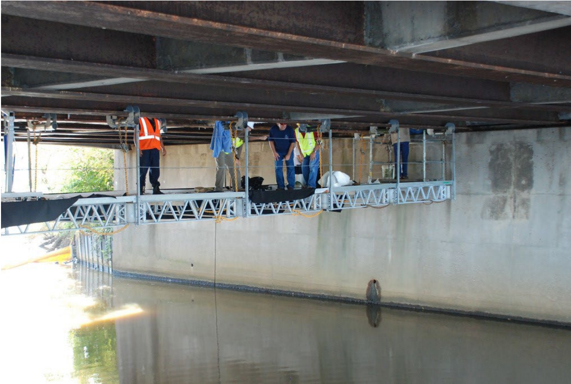
Figure 10. Example of temporary scaffolding hanging underneath a bridge.
