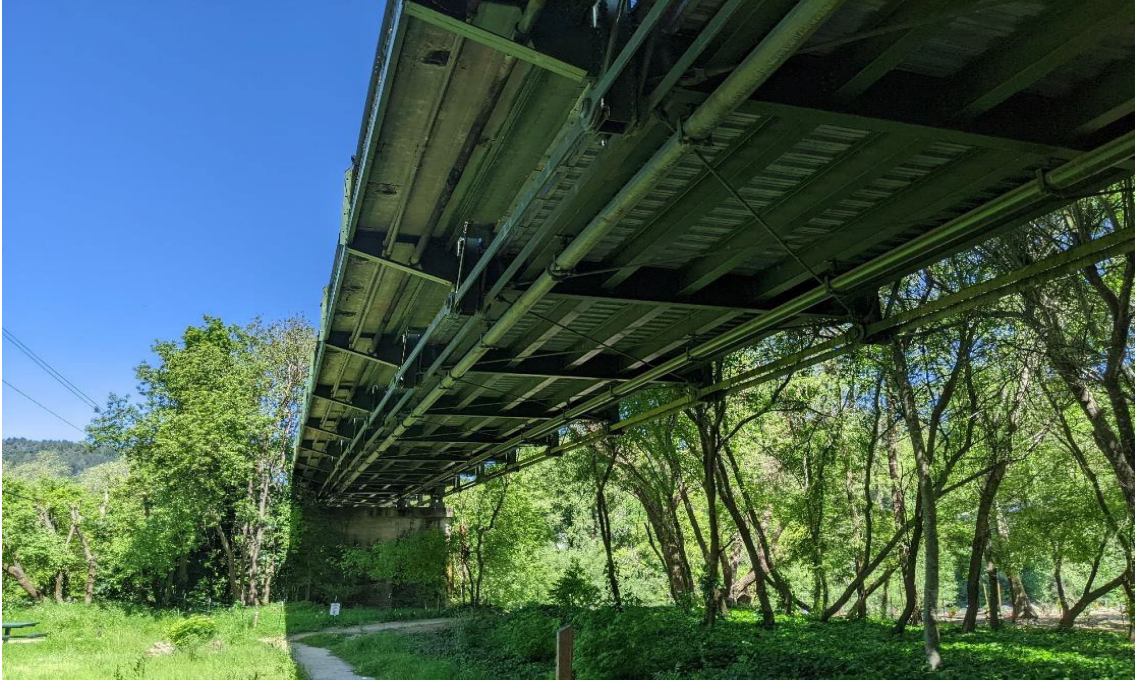
Figure 9. Looking northwest under the Guerneville Bridge at the existing Beanwood Force Main hanging on the underside.
