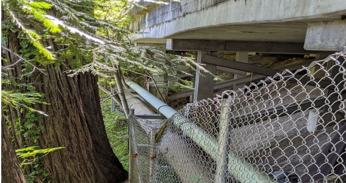
Figure 14. The existing 16-inch diameter steel Main Force Main and 8-inch diameter gravity sanitary sewer suspended along the Hwy 116 viaduct.
