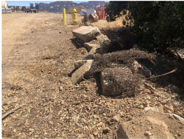
Example of wire meshing and concrete features uncovered during trenching 8/25/23.
