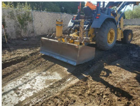
Archaeological monitoring of grading within modular footprint on 9/22/22.
