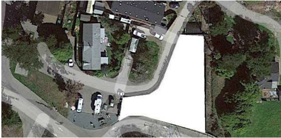
Site 2: San Simeon Campground Staff Housing.
