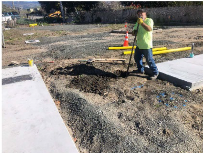
Excavations for bollards in modular footprint previously disturbed area 1/27/23.
