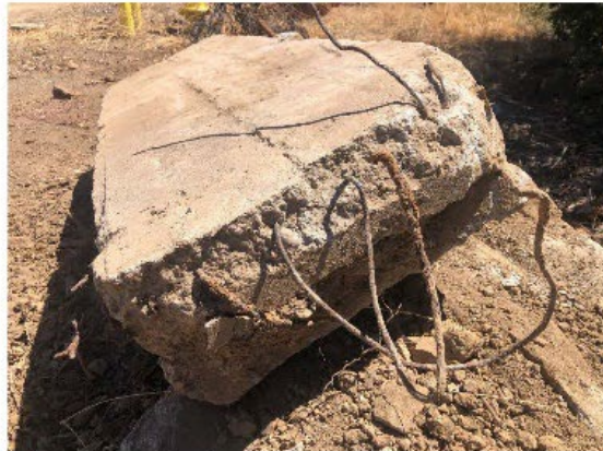
Concrete rubble from the animal enclosures from Hearst-era zoo at Elephant Hill, showing double rebar cages. The concrete was buried at 24-36" below the surface.
