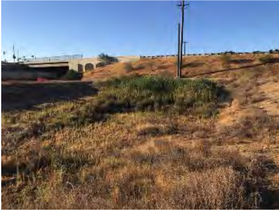
Photo 1. Overview of Feature 1 (F1). Area is between a berm adjacent to the railroad track/Interstate 215 (I-215) and commercial property. Photo taken facing south. June 27, 2018
