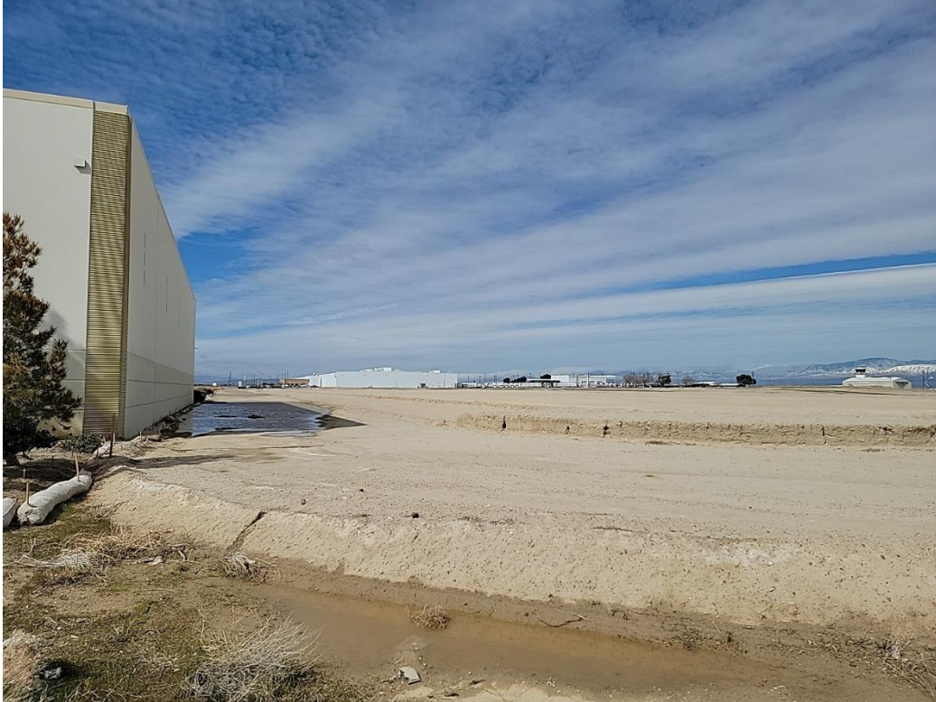
Photograph 3: View of the southeast corner of the project site, looking west.
