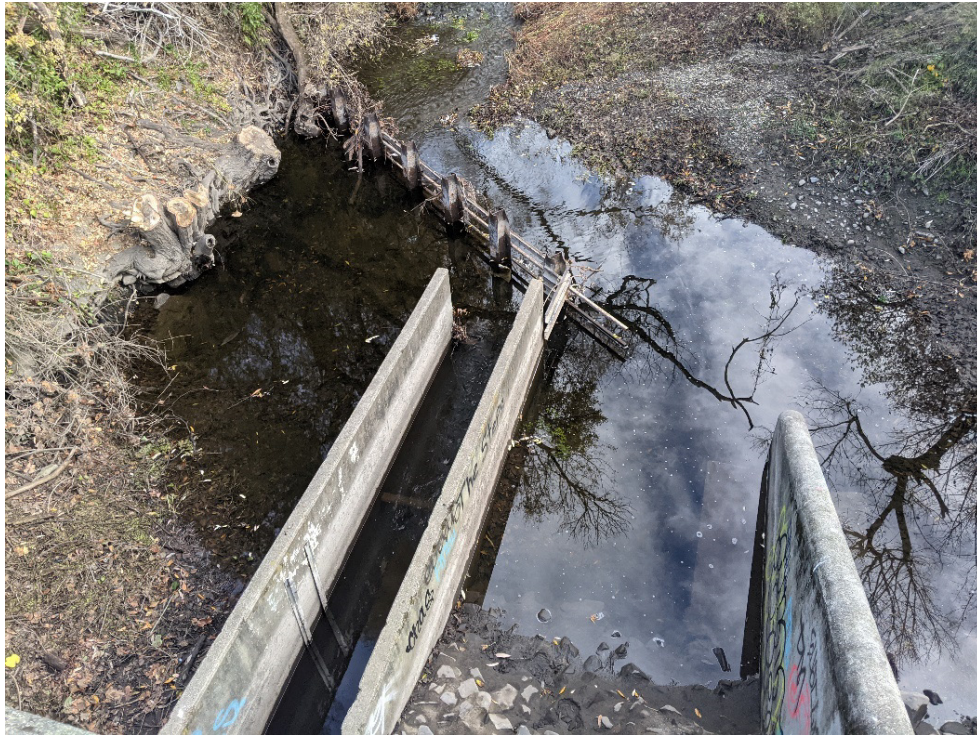
Photograph 2.2-2. Aerial View of E Street Bridge Fishway Extension Site.
