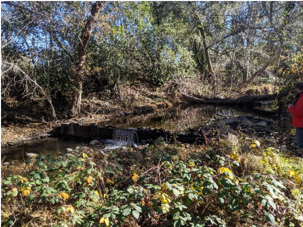
Melita Diversion Dam, Looking East
