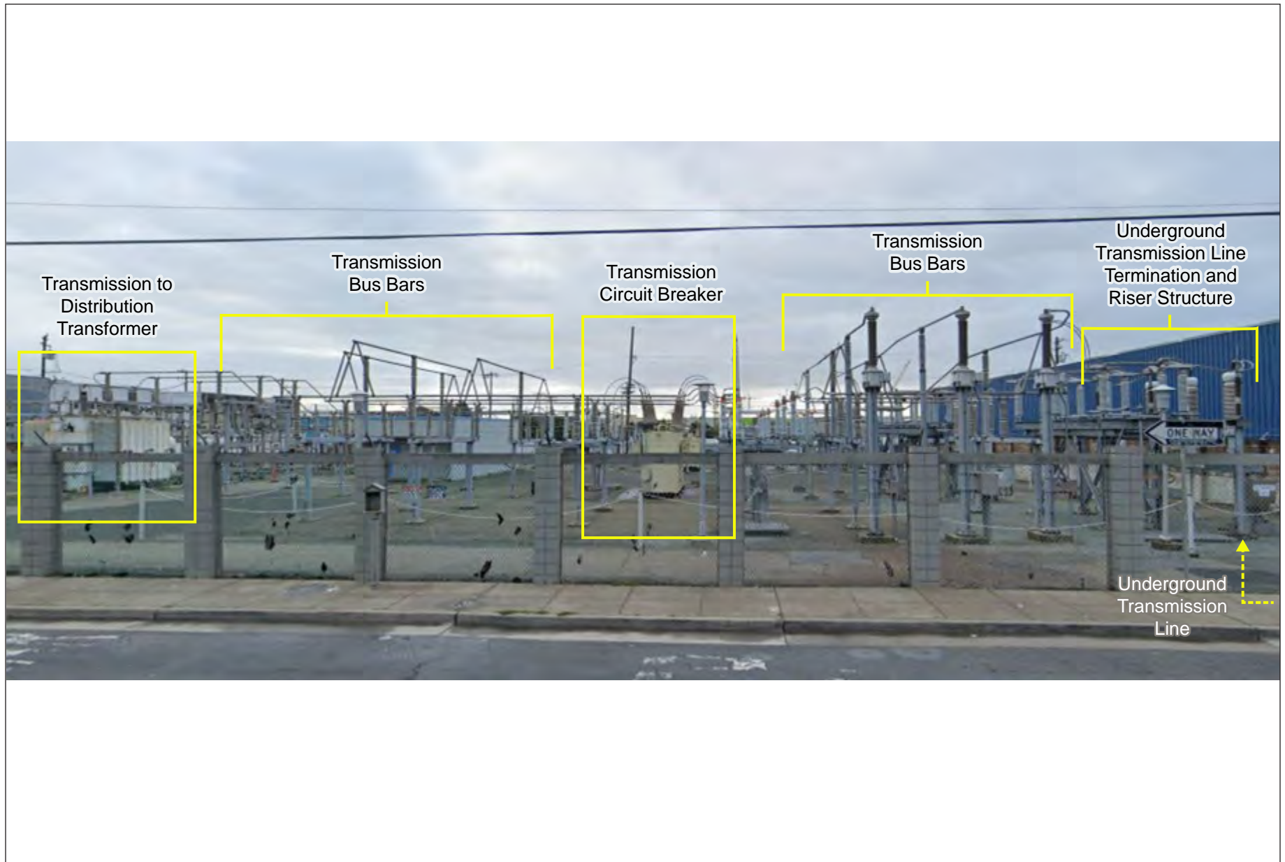
Figure 3 Examples of Above-Ground Infrastructure at an Electrical Substation
