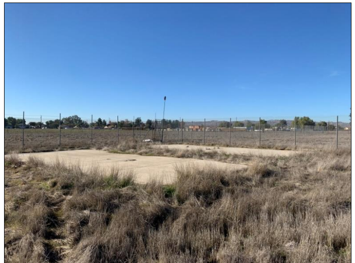
6. Small concrete foundations on the south central portion of the northern parcel, view facing
