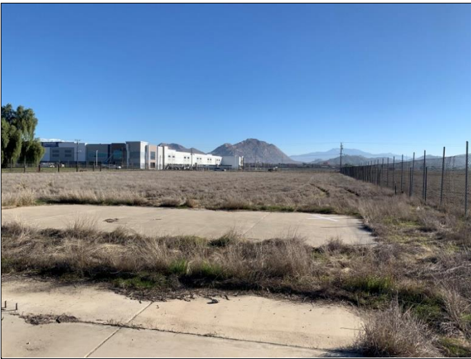
9. Concrete foundation on the south central portion of the northern parcel, view facing east.
