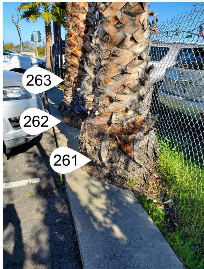
Figure 4. These co-owned palms are growing over the existing concrete curb, preventing them from properly anchoring into the soil. These palms should be removed due to their hazardous condition. Removal will require the neighbor's permission.
