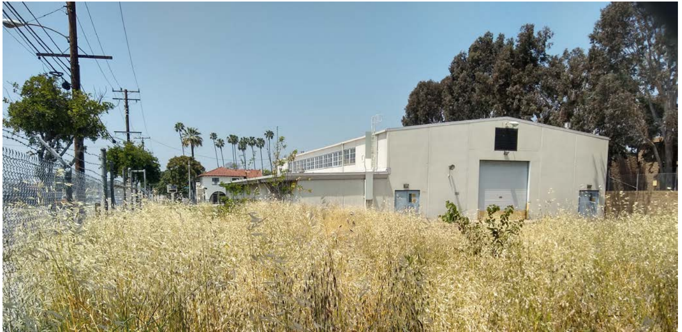
Photo 4. Montebello Armory, south and east façades. Ascent 2023.
