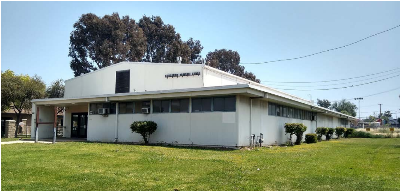
Photo 1. Montebello Armory, west and south façades. Ascent 2023.
