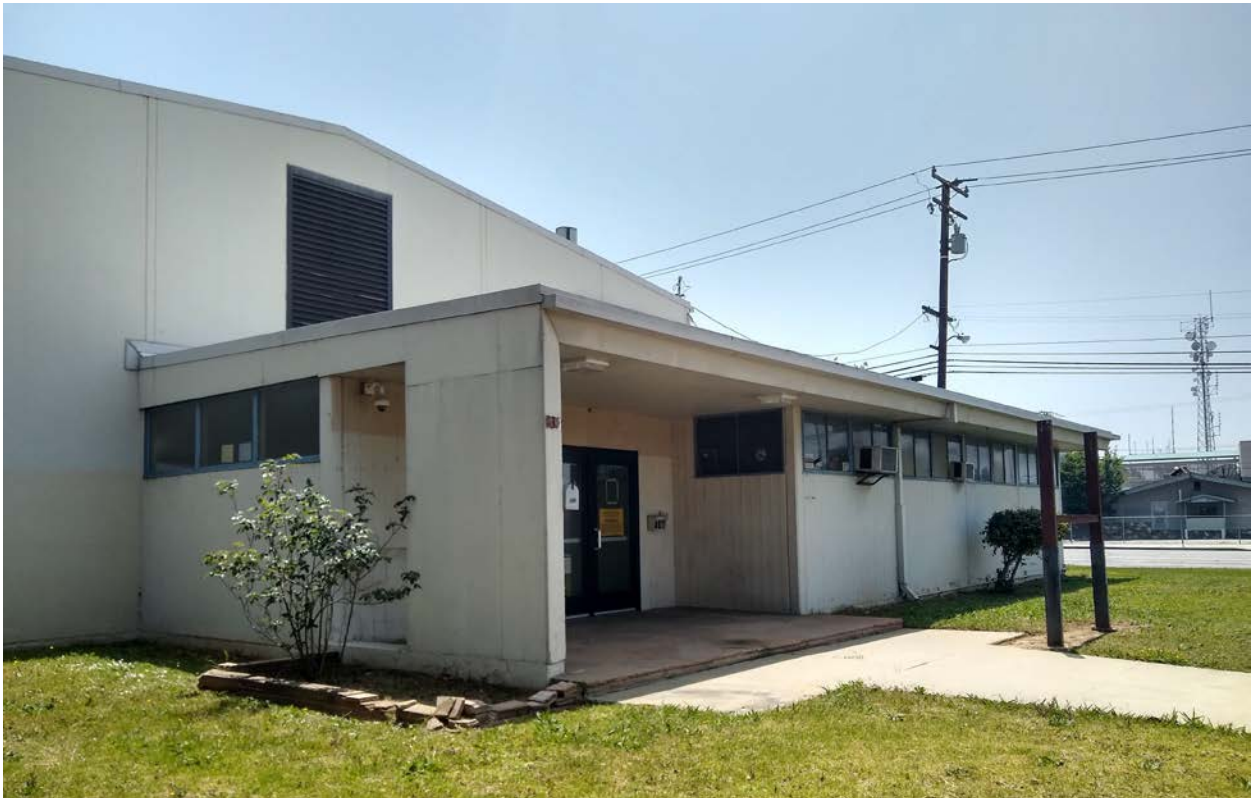
Photo 2. Montebello Armory, west façade, main entry. Ascent 2023.
