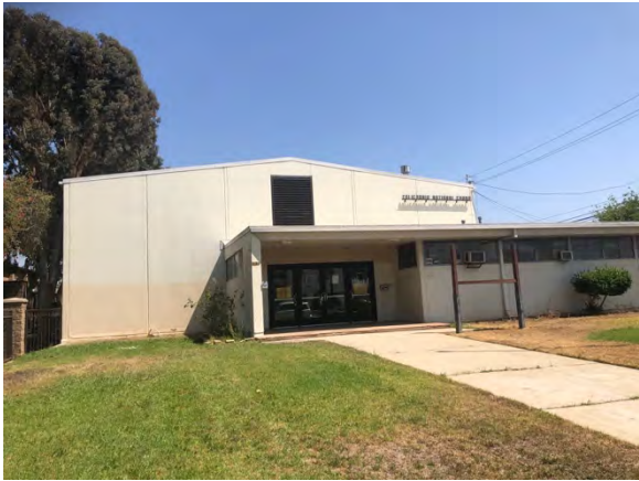
Eastern view of the Subject Property from George Hensel Drive.
