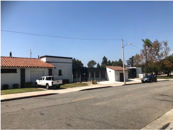
Northwest view from the Subject Property towards the aquatic center and City Park.
