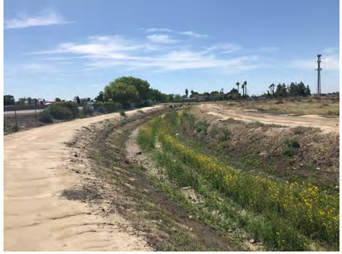
View of Peoples Ditch and barren areas, facing west. April 27, 2020.
