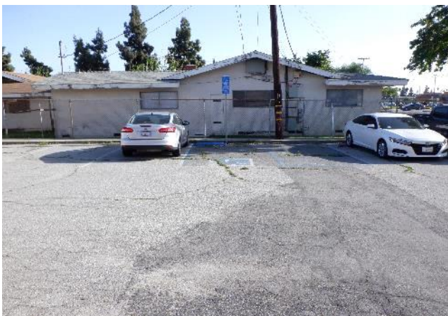
Photo 4: 578-580 N. Azusa Ave, N elevation, looking S
