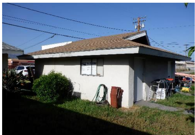
Photo 7: Ancillary building, W and S elevations, looking NE
