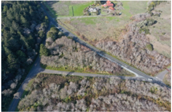
The Project site looking from above (drone image).
