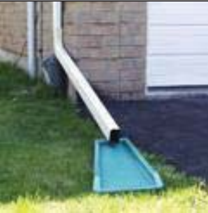
Simple Downspout Dispersion Source: toronto.ca/environment/water.htm
