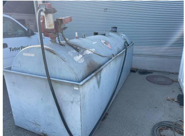
Photo #10 View of 1,000-gallon diesel fuel tank and suspected oil/water separator on northern portion of central-northern warehouse.
