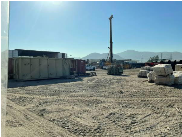
Photo #45 View of stored materials on southern portion of site.
