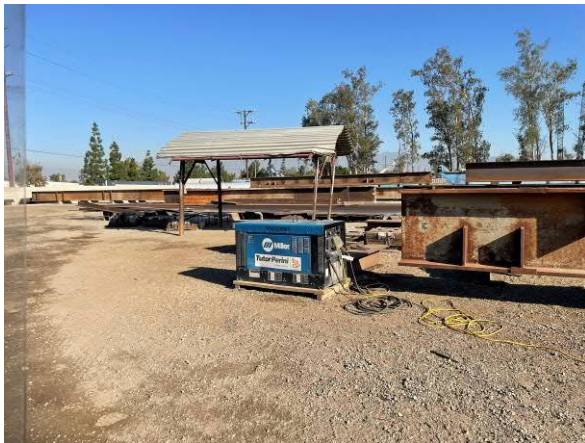
Photo #39 View of generator on central-southern portion of site.
