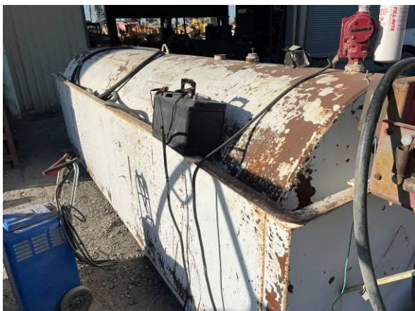
Photo #11 View of additional 1-000 gallon diesel fuel tank on northern portion of central-northern warehouse.
