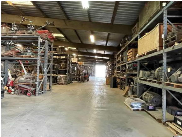
Photo #19 View of interior of warehouse on northeastern portion of site.
