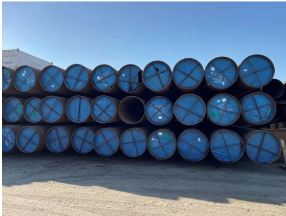
Photo #31 View of steel pipe storage on central portion of site.
