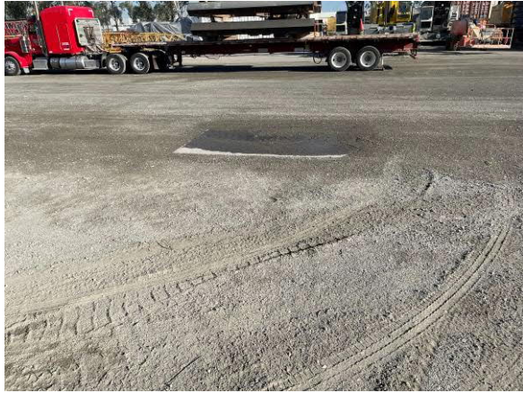
Photo #13 View of concrete pad with manhole cover, possible location of former UST.
