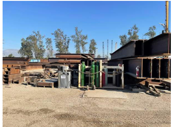
Photo #38 View of compressed gas storage on central-southern portion of site.
