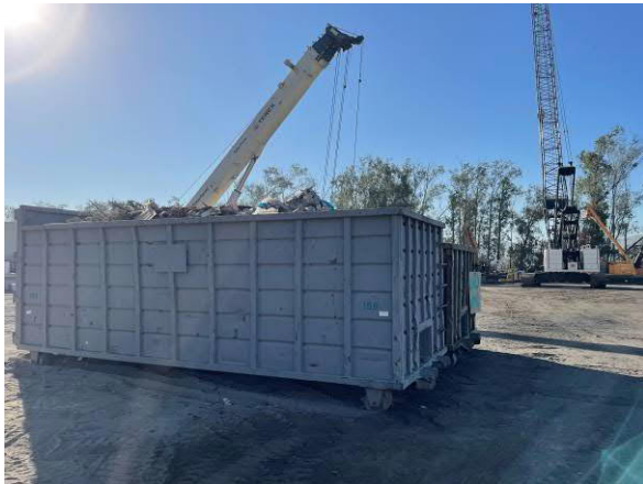
Photo #25 View of solid waste dumpsters on northeastern portion of site.
