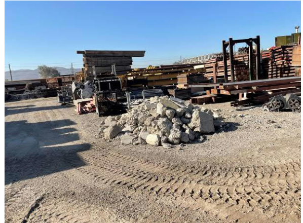
Photo #44 View of concrete debris on central-southern portion of site.
