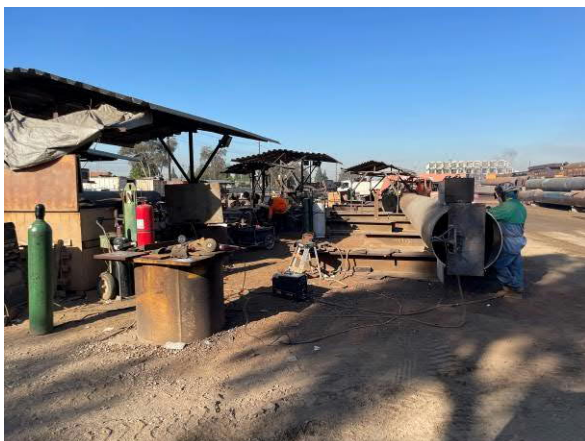
Photo #35 View of maintenance area on central portion of site.
