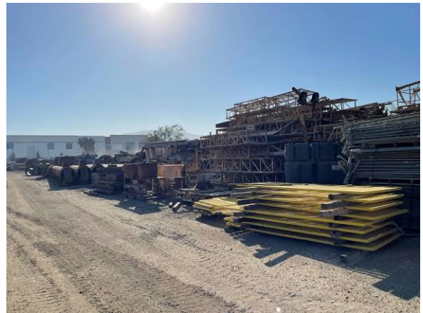
Photo #34 Additional view of materials storage on central portion of site.
