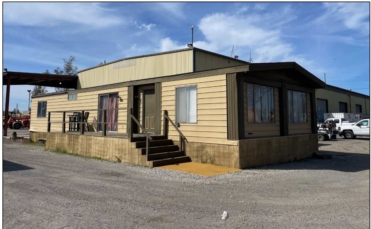
Figure 5-4. Overview of modern manufactured building (Building 3) (foreground) with Building 1 in background, facing southwest
