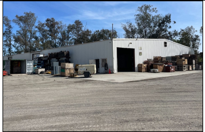
Fig 2: Overview of modern warehouse (Building 2), facing NE
