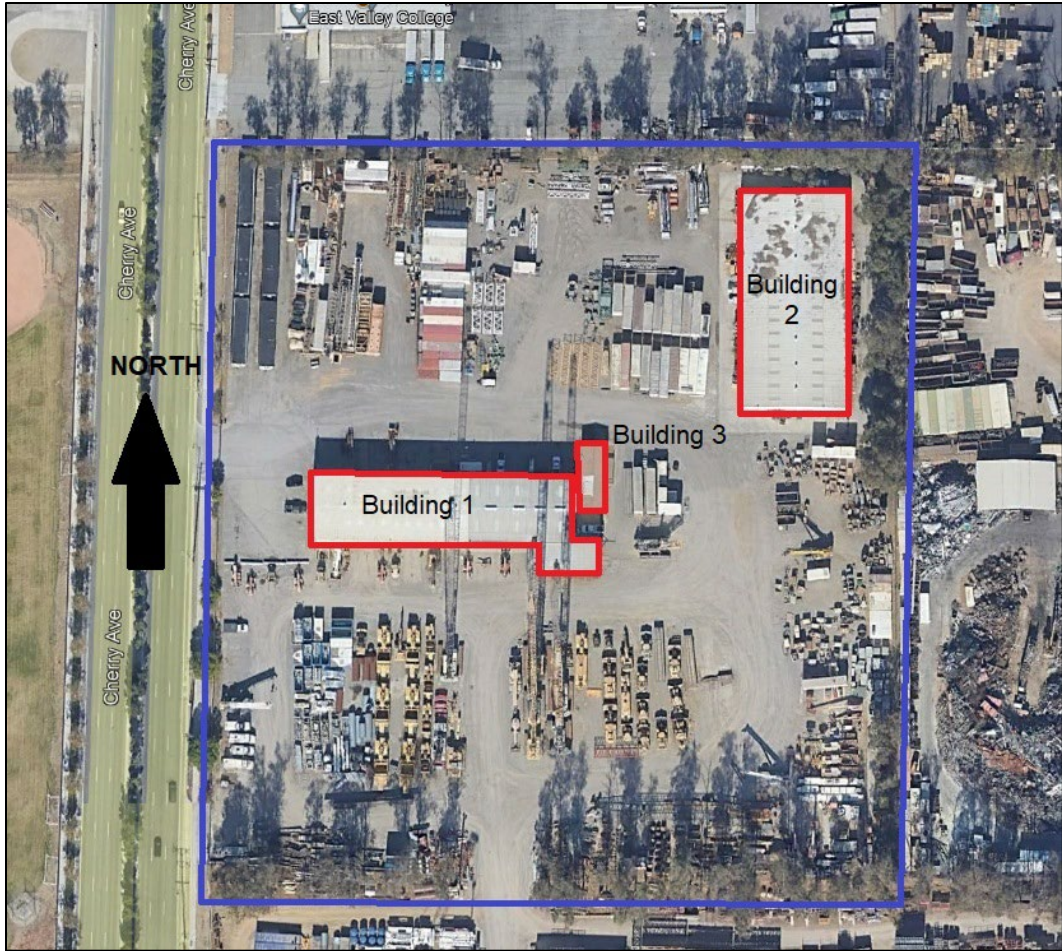
Figure 5-1. APN 023-619-114 showing historic and modern buildings on property.
