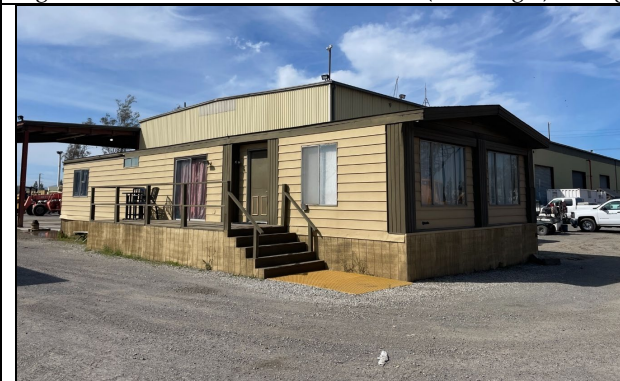
Fig 3: Manufactured building (Building 3), facing SW
