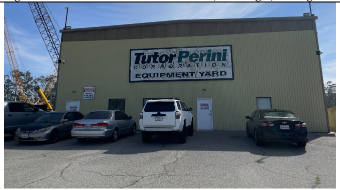
Fig 4: West elevation of Building 1, facing east
