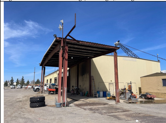
Fig 5: Covered work/storage area SE of Building 1, facing W
