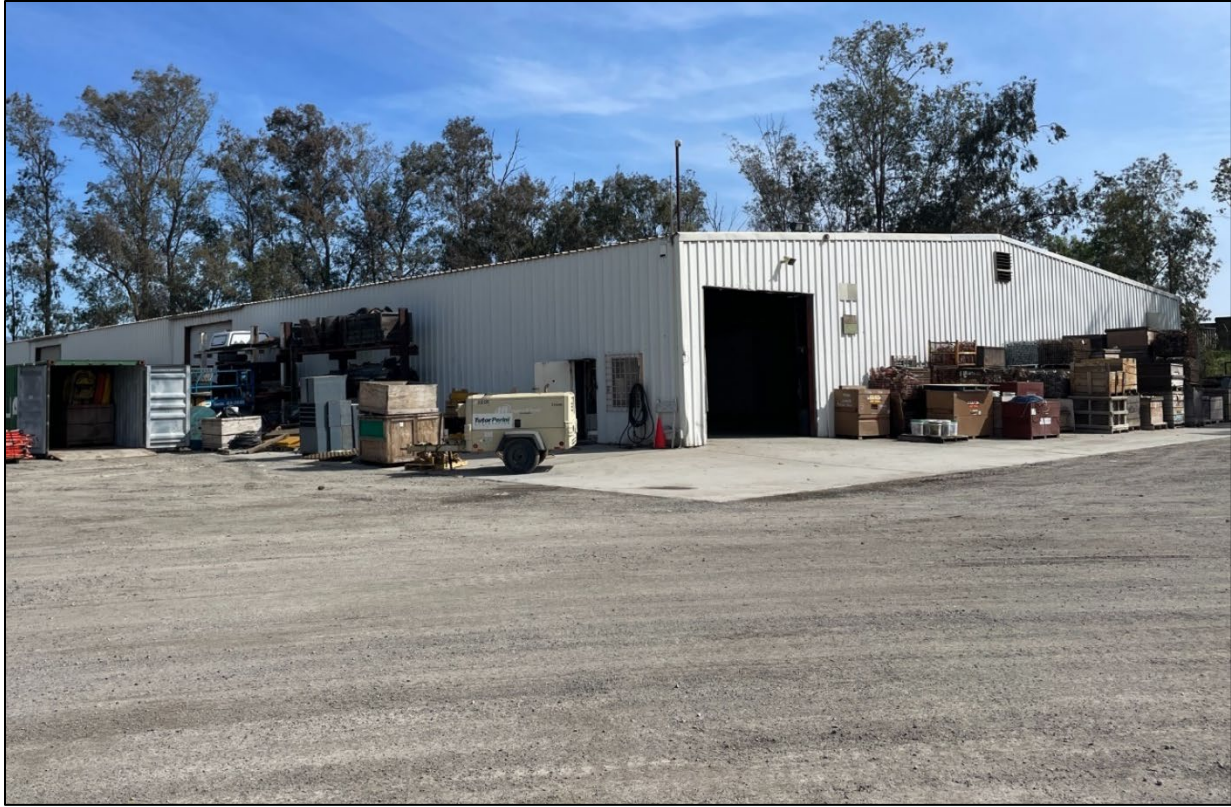
Figure 5-3. Overview of modern warehouse (Building 2), facing northeast
