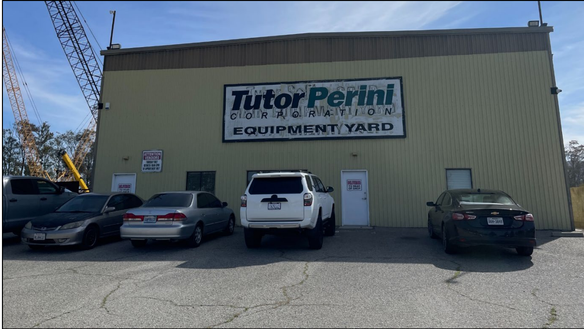
Figure 5-7. West Elevation of Building 1 at 11171 Cherry Avenue, facing east
