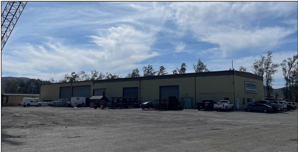
Figure 5-2. Overview of historic warehouse (Building 1), facing southeast
