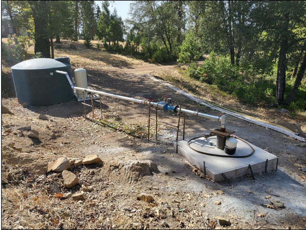
Photo 3. Overview of existing test well and associated infrastructure.
