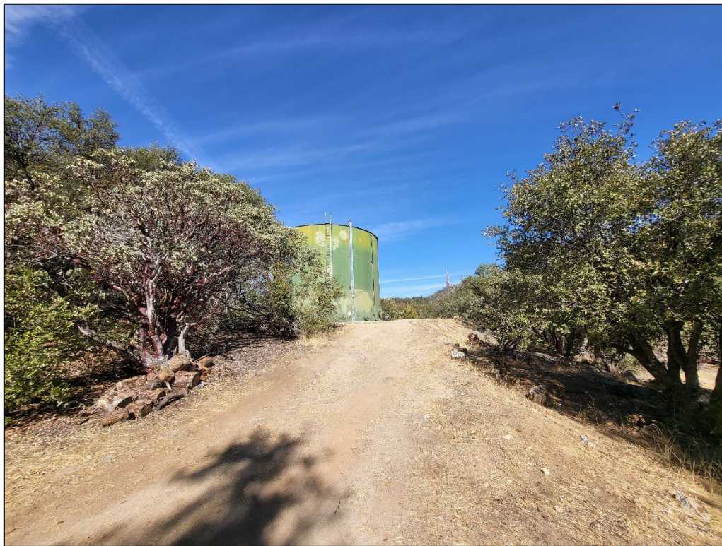
Photo 4. Overview of dirt access road/access to existing water storage tank in eastern portion of project area.
