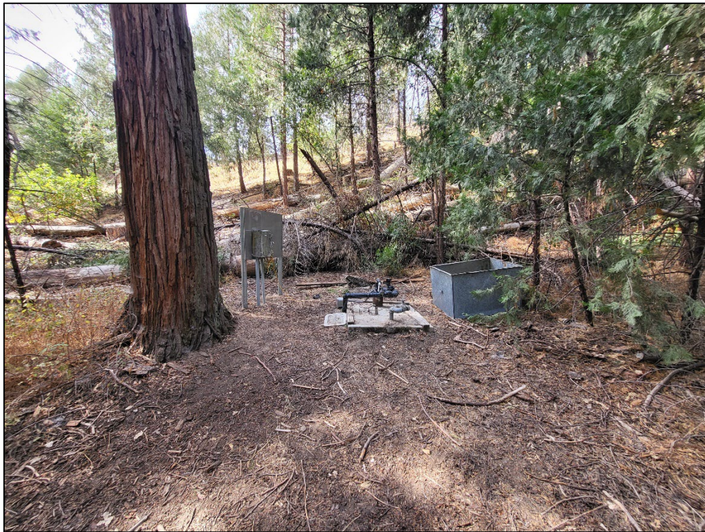
Photo 14. Overview of existing Well No. 2 proposed for improvements.
