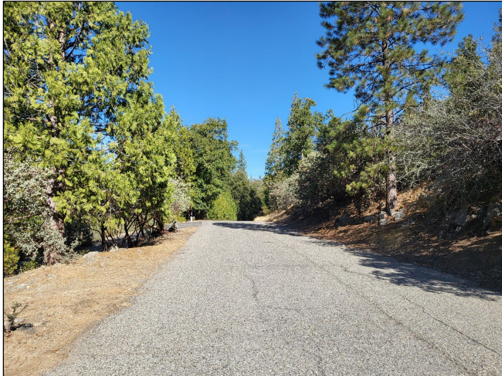
Photo 8. Overview of transmission pipeline location in existing road (Teaford Poyah), where the mixed oak pine and woodland transitions into mixed conifer forest.
