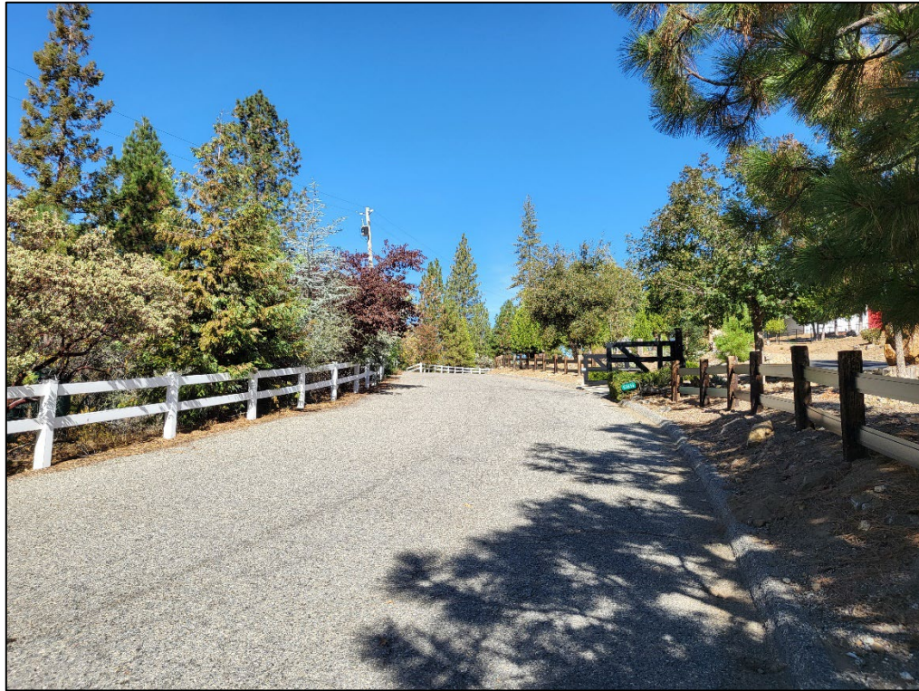
Photo 7. Overview of transmission pipeline location in existing road (Moic Drive).
