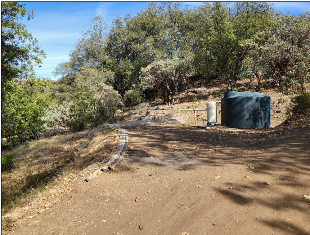
Photo 2. Overview of proposed generator and electrical panel improvement adjacent to existing test well. Surrounded by mixed oak and pine woodland.
