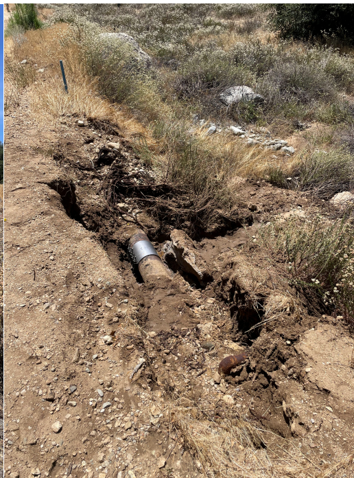
Pipeline to be Abandoned - SW View
