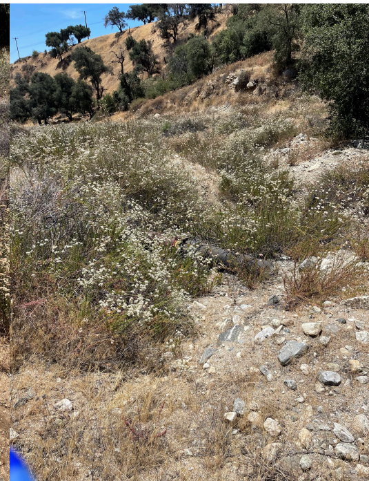
Pipeline to be Abandoned - SW View
