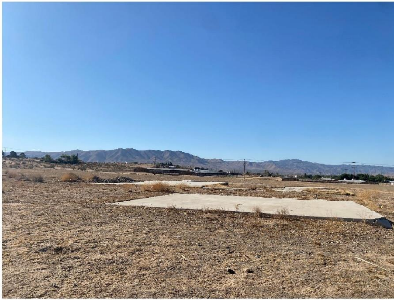
Figure 10: Overview of concrete foundations in the southeast quarter of the Project, view north.
