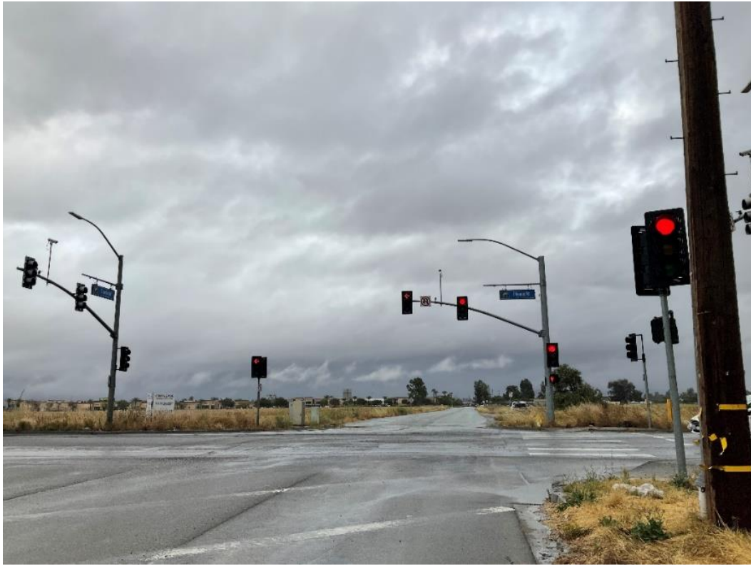
Figure 5-5. Northern extent of Trumble Road from intersection with Ethanac Road, facing north.
