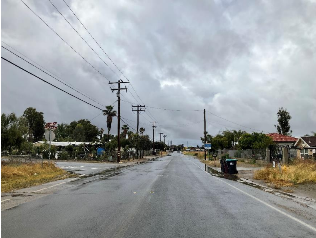
Figure 5-9. Overview of Sherman Road from northern extent at intersection with Harris Avenue, facing south toward Ethanac Road.
