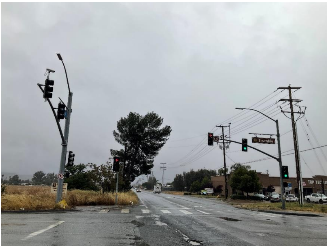
Figure 5-7. Improvements made at intersection of Ethanac and Trumble Roads, facing east.
