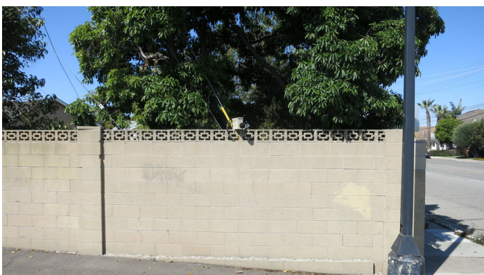
Noise Measurement Site L1 - looking west
