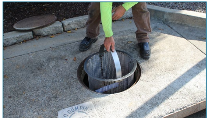
Easily removed without entry into basin.
