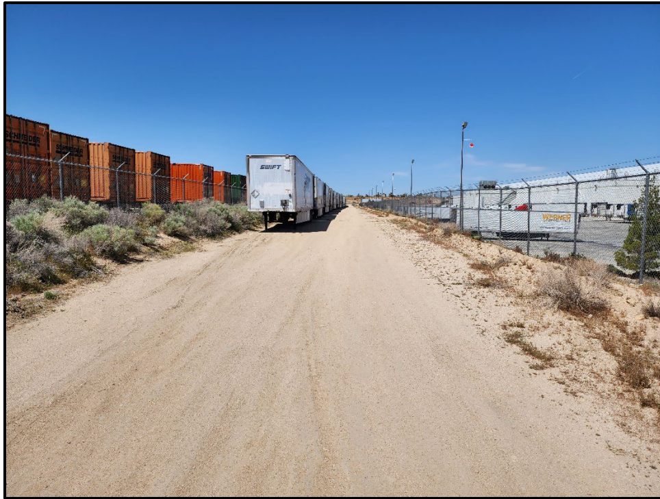
Plate 4.2–3: Overview of the panhandle driveway, facing west towards Enterprise Way.
