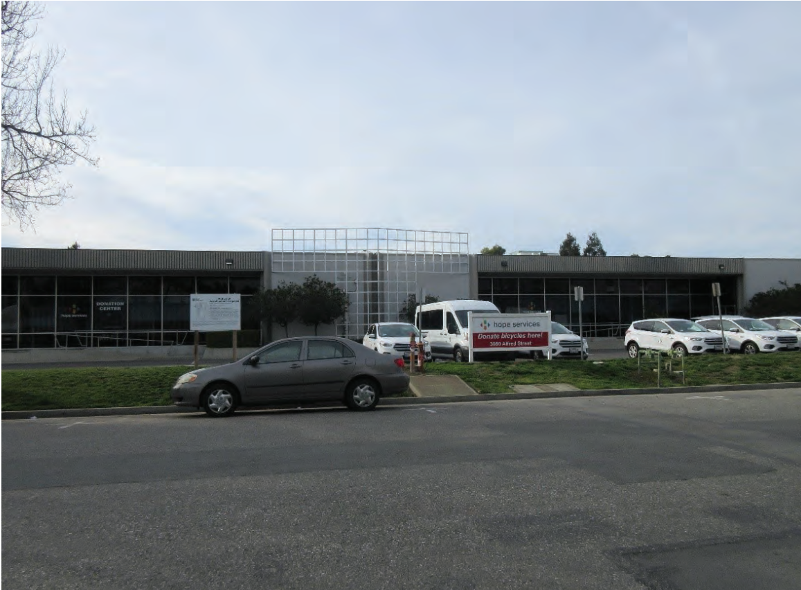
Photo 1: View of the on-site 3080/3100 Alfred Street building (MCA-3) looking west.
