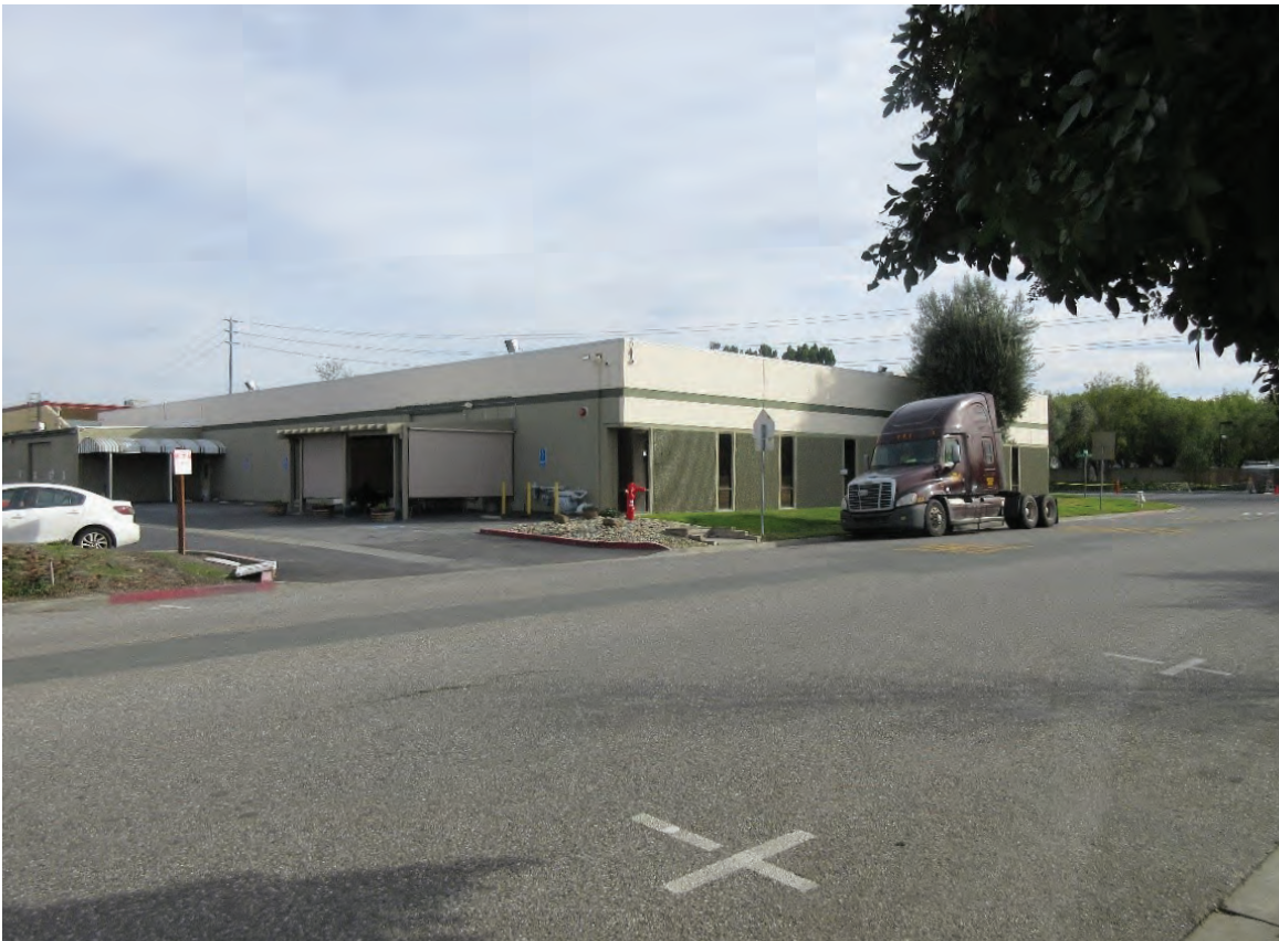
Photo 6: View of industrial building on Alfred Street, looking south toward Space Park Drive.
