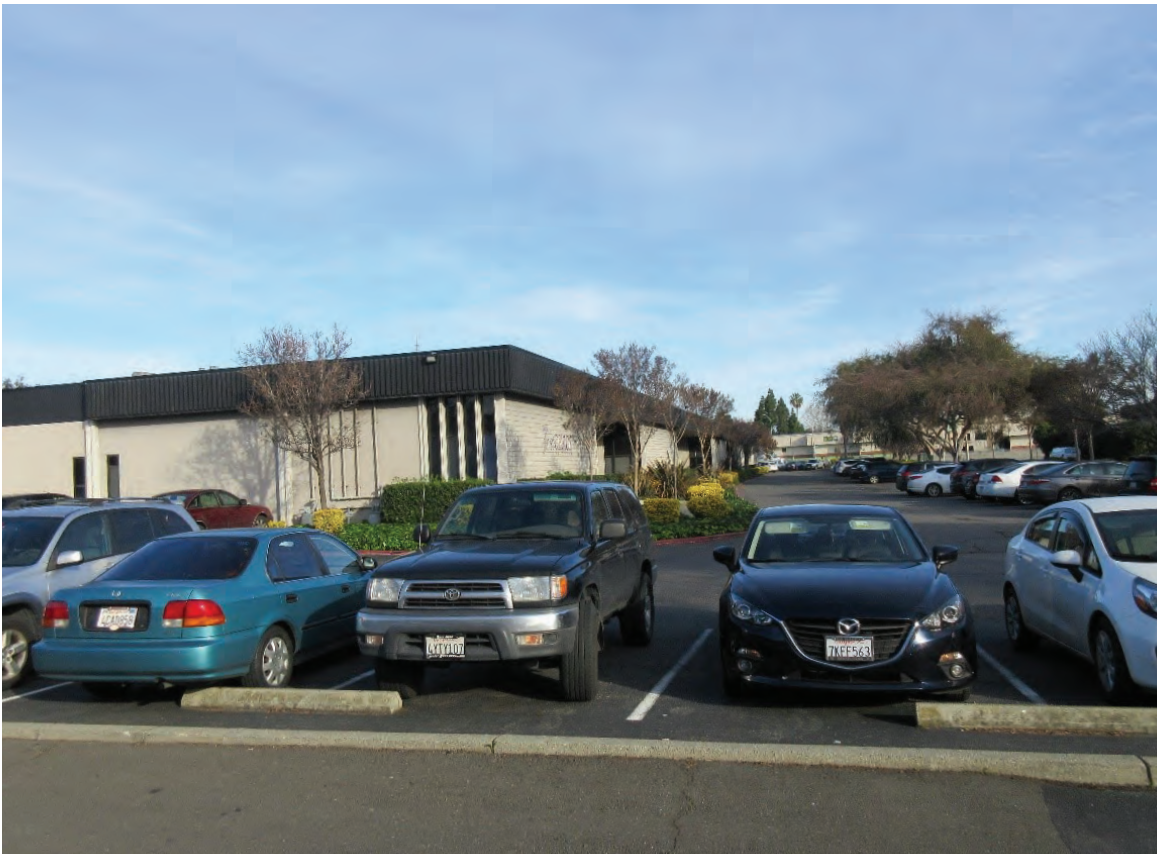
Photo 4: View of the commercial building to the north of the MCA-3 building on Alfred Street.
