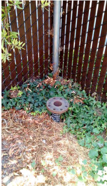
Photo 13: Western fence line near the southwest corner of the site - bump-out in the fence that appears to have been an enclosure for some kind of equipment, with a pipe flange sticking up out of the ground.
