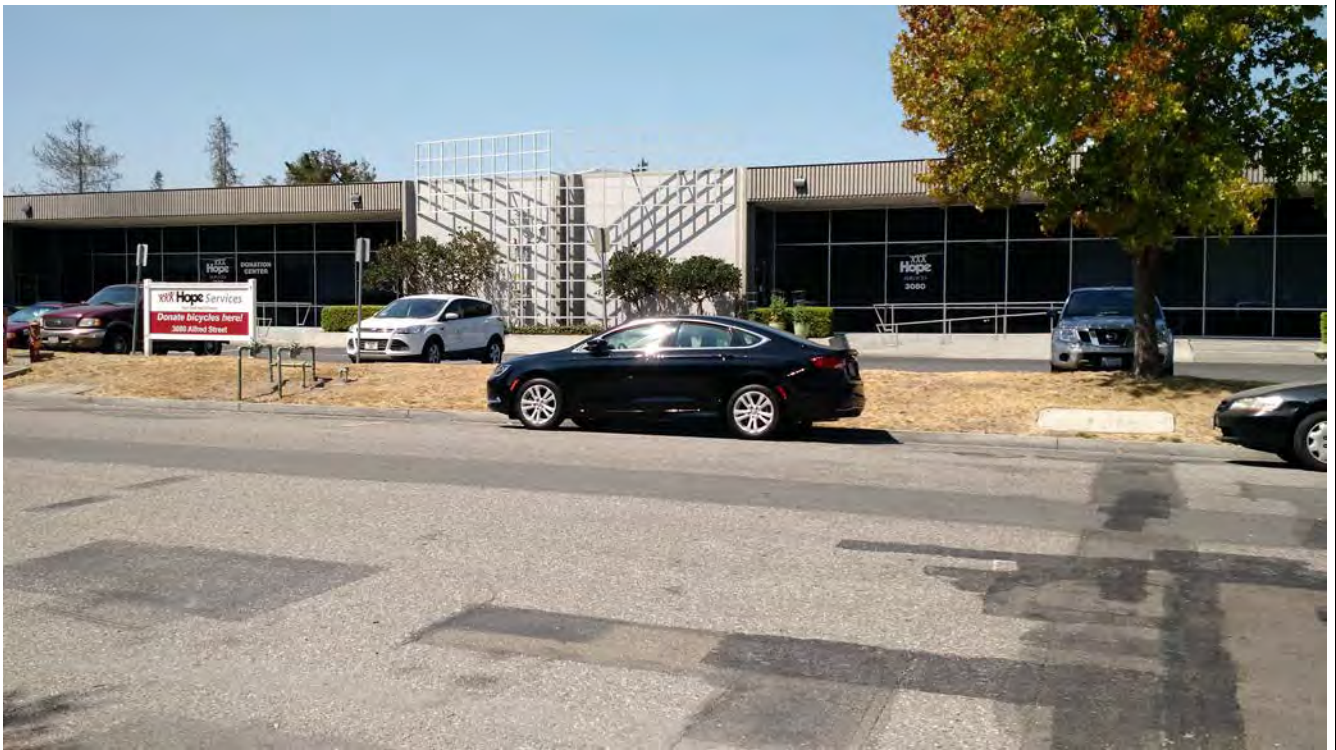
Photo 1: Front of the site building at 3080/3100 Alfred Street, with the 3100 side of the building on the left and the 3080 side of the building on the right. Photograph facing west.
