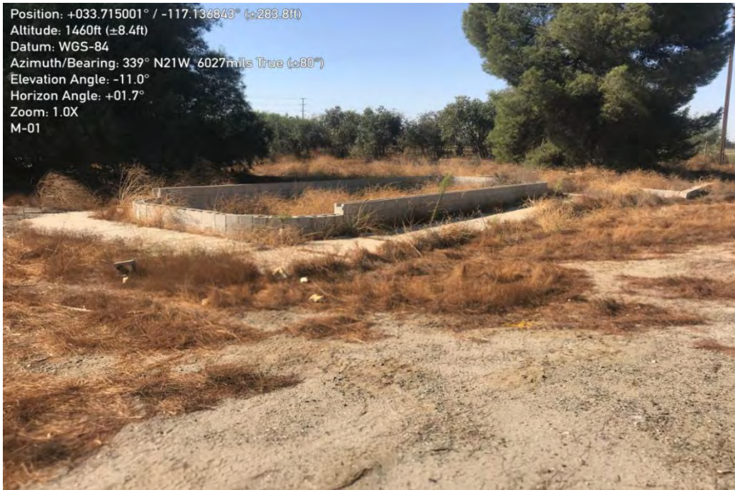
Photo 1: Northwest view of basin feature M-01 bordered by block walls.
