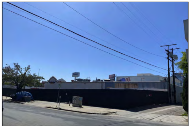
View 4: From the east side of Westgate Avenue, looking southwest at the Project Site.
