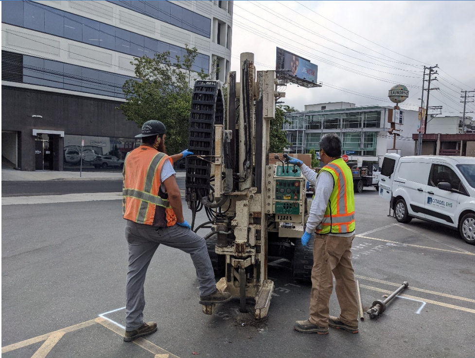
PHOTO 1: Drilling operations at B2 (6/21/21).
