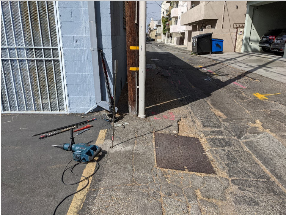
PHOTO 4: Installing boring B7 with the Roto-Hammer Drill (6/22/21).
