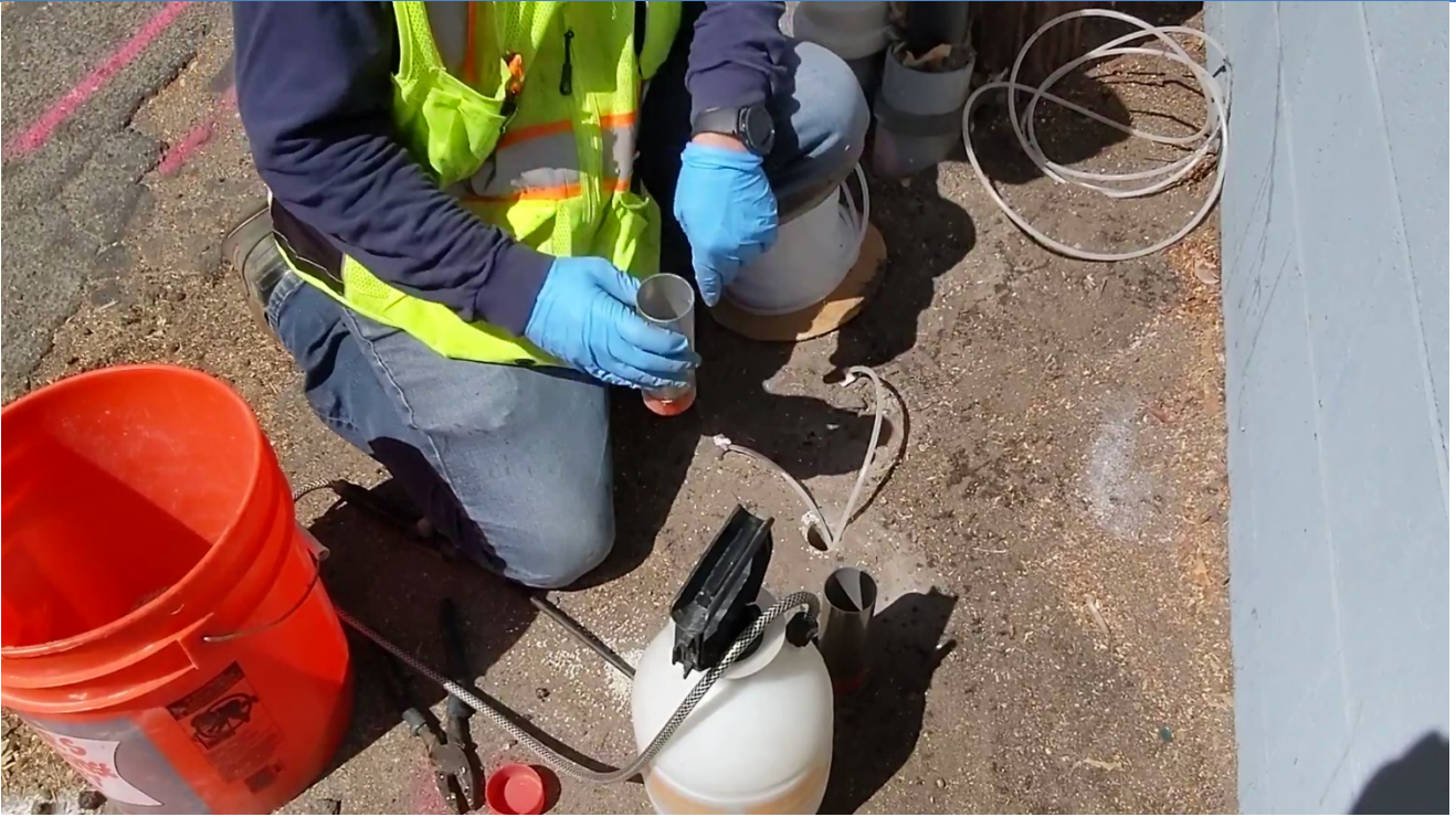
PHOTO 5: Installing vapor probes in boring B5 (6/21/21).
