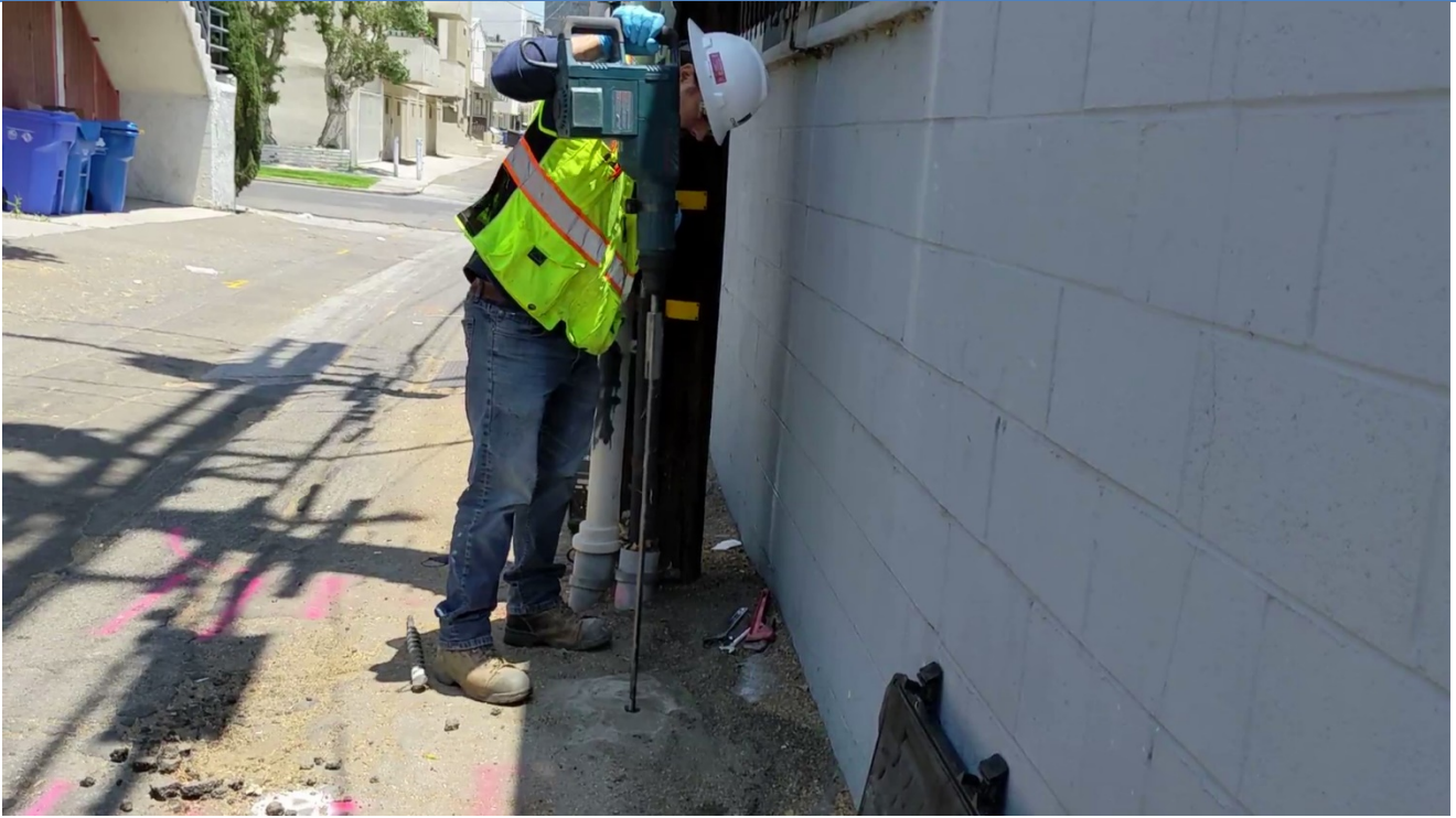
PHOTO 3: Installing boring B5 (6/21/21).
