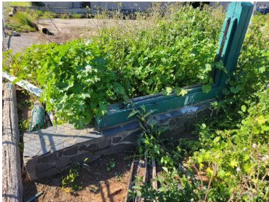
Front signage and mailbox area now in disrepair and overgrown.
