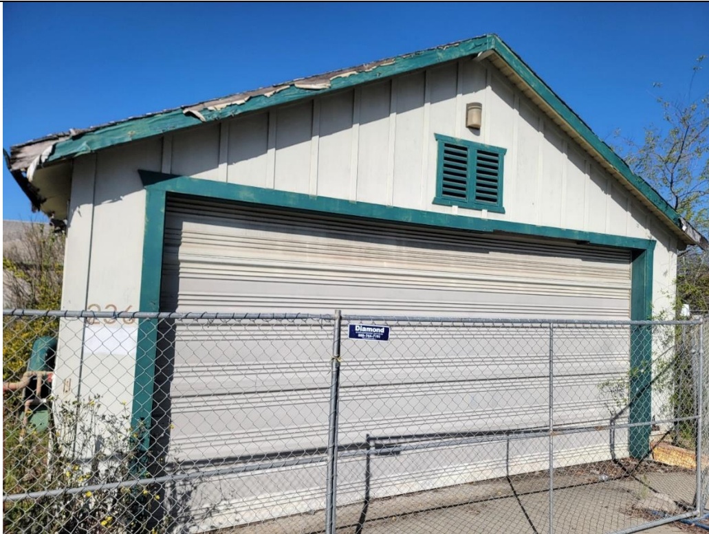
Photograph 8: Garage, east elevation, modern garage door.
