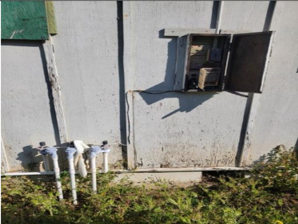
Photograph 6: Barracks, south elevation, modern irrigation system.
