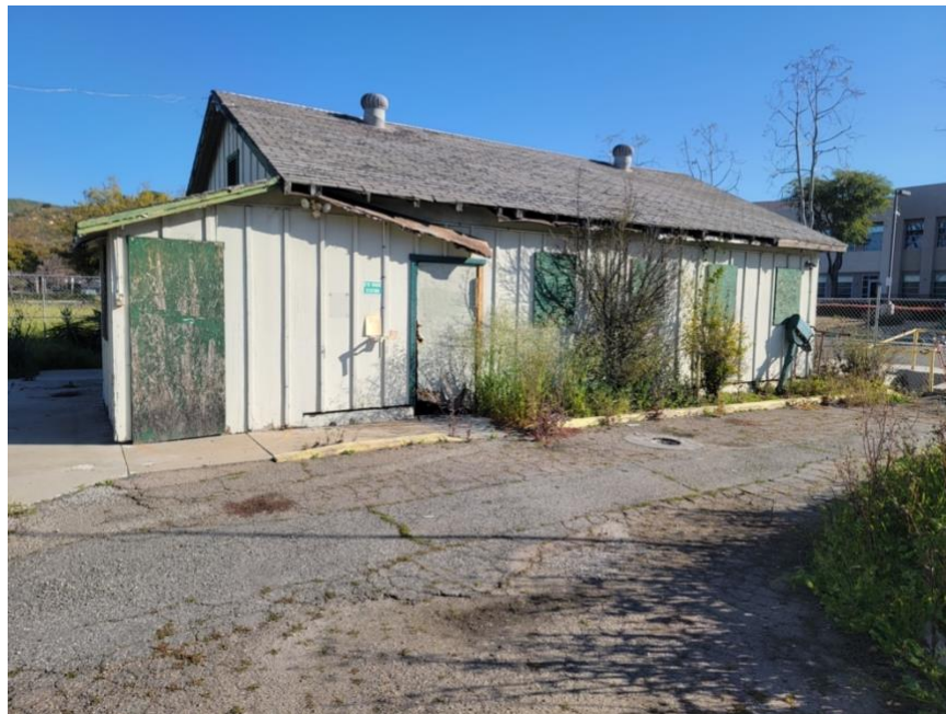
South entrance to Garage. Modern surface-mounted eye wash station visible.
