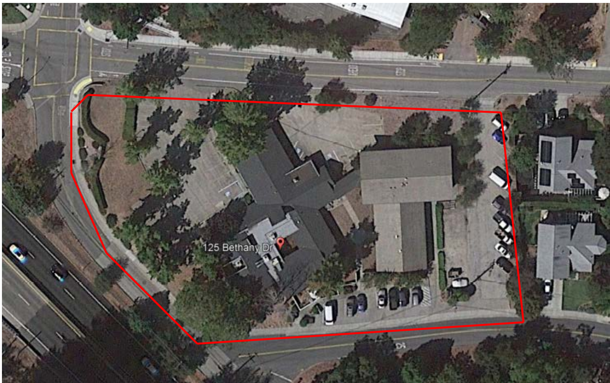
Image #1 –Project area bordered by Tabor Drive, top of image, Scotts Valley Drive, to left and Bethany Drive, bottom of image.
