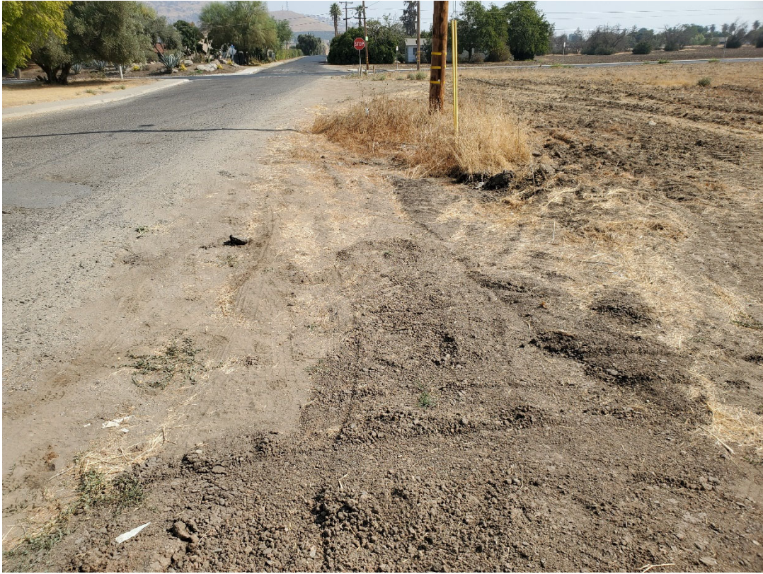
Photograph of Basin 1 taken facing east on October 21, 2020.
