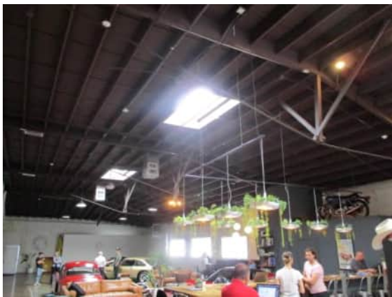
Photo #5: Showroom and ceiling detail
