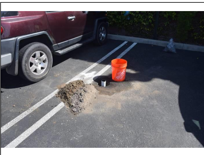
17. Newly drilled monitoring well on northwestern portion of the subject property
