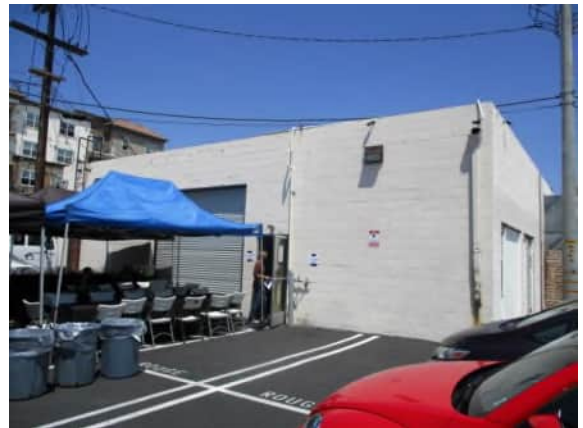
Photo #30: 4130 West elevation
