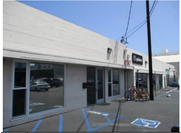
Photo #32: 4130 West elevation
