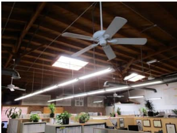
Photo #53: Office cubicles and ceiling detail
