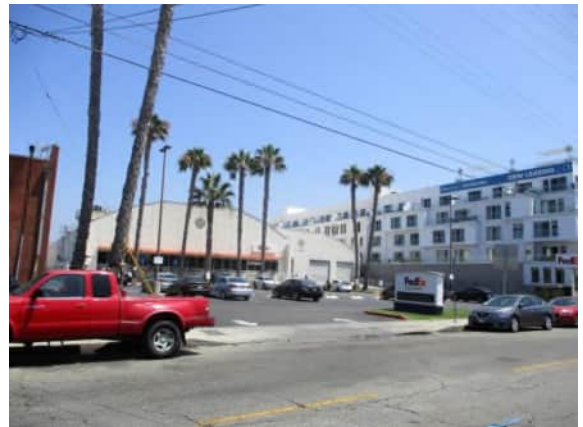
Photo #60: South adjacent FED EX
