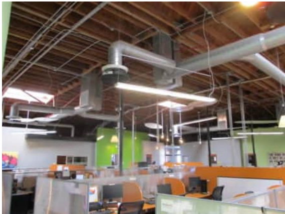
Photo #51: Office cubicles
