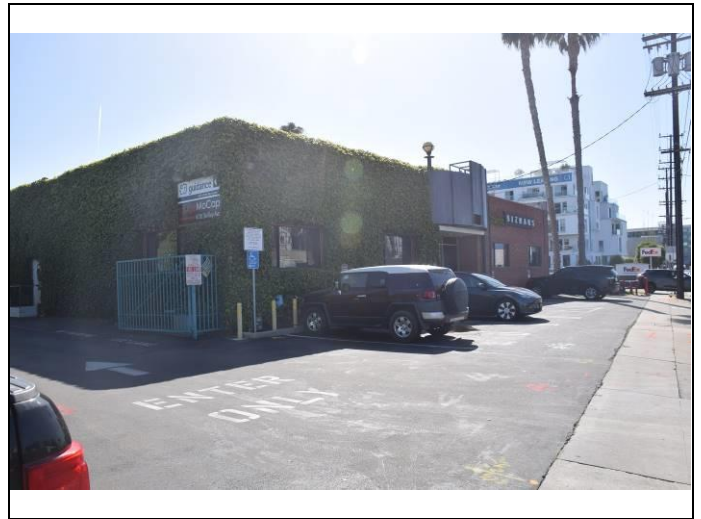
2. Southwestern corner of the subject property
