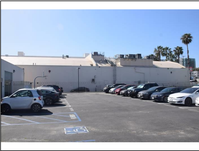
7. Southern side of the subject property
