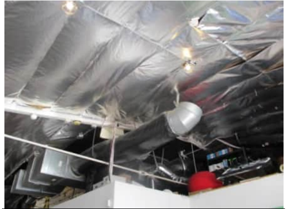
Photo #14: Ceiling detail
