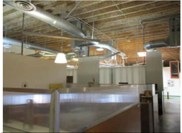
Photo #38: Office cubicles
