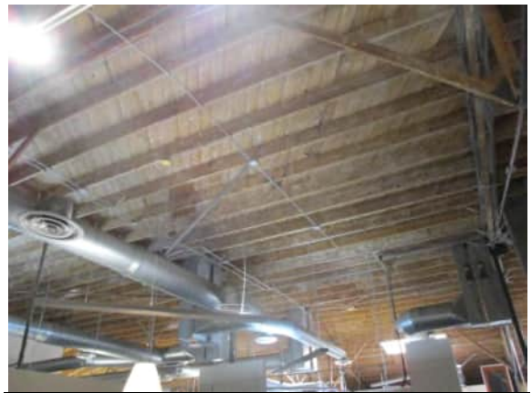
Photo #36: Ceiling detail and HVAC vents
