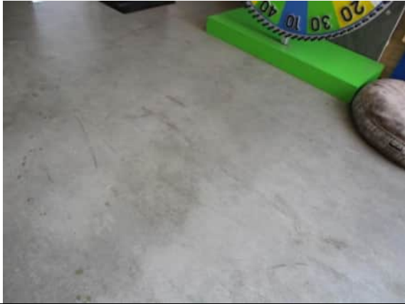
Photo #13: Floor detail
