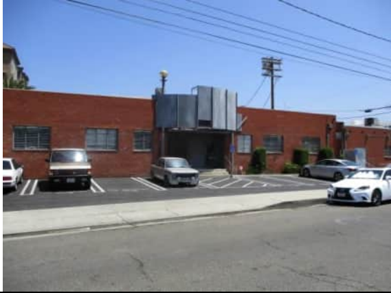
Photo #1: Front view of Subject Property (4112 Car Club) as viewed from Del Rey Avenue
