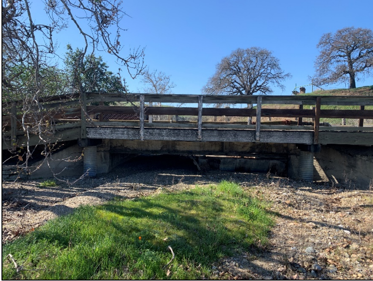
Photo 5: Photo of existing bridge on Arroyo Road in the BSA, looking east from the Dry Creek channel.
