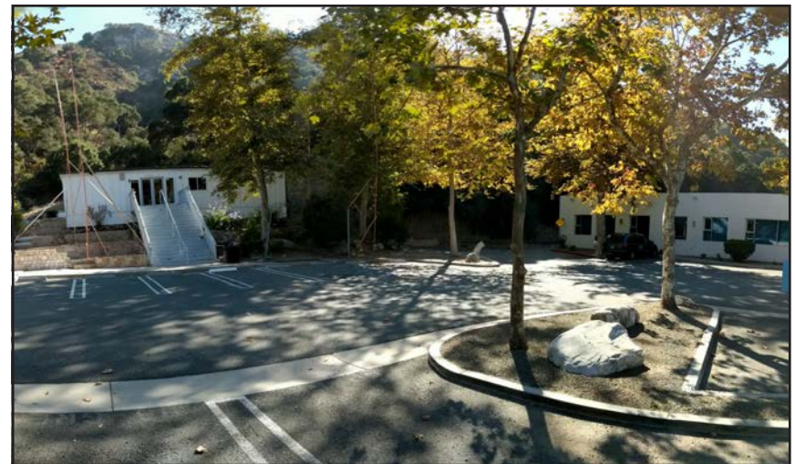
View 4: Views of Building C and B.
