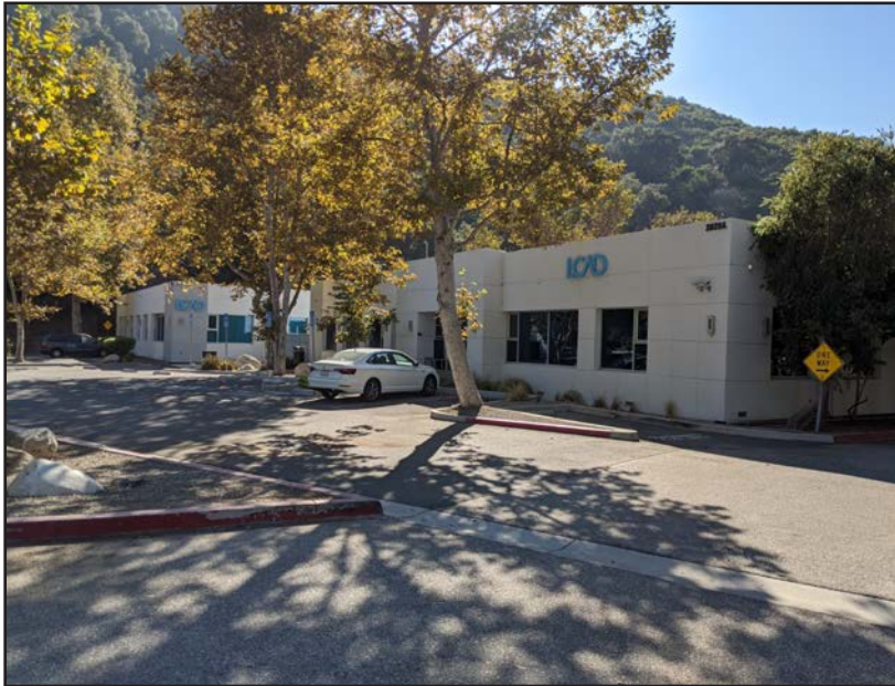
View 1: Views of Buildings A and B.
