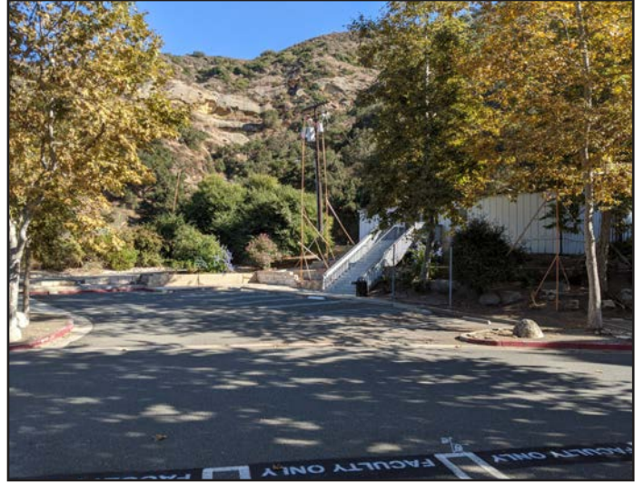
View 6: View of Building C Looking East.
