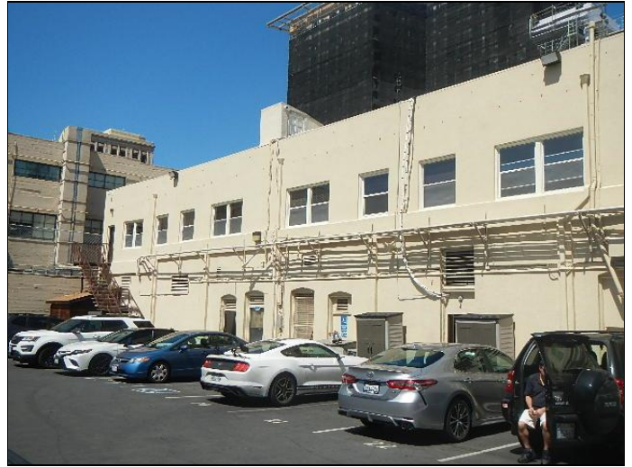
2. Parking and rear façade of 2128 building
