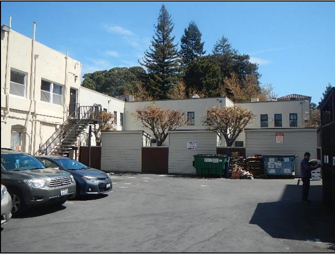
1. Parking and rear façade of 2128 building
