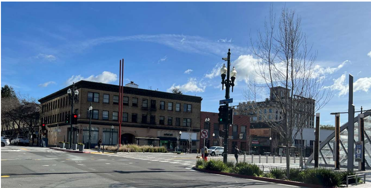
Figure 9 View of the Shattuck Avenue Commercial Corridor Historic District, Eastern Side of Shattuck Avenue, 2161 Shattuck Avenue (L), View East
