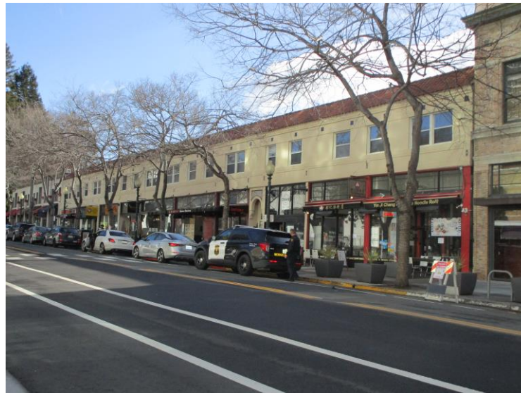
Photograph 1. View of Thomas Block Building, facing east. Photo taken January 19, 2023.
