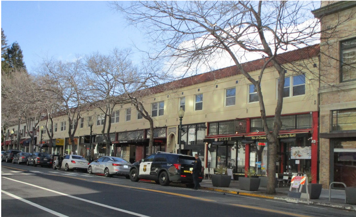
Photograph 3. View from Center Street looking south at the 2132-2154 Center Street building.
