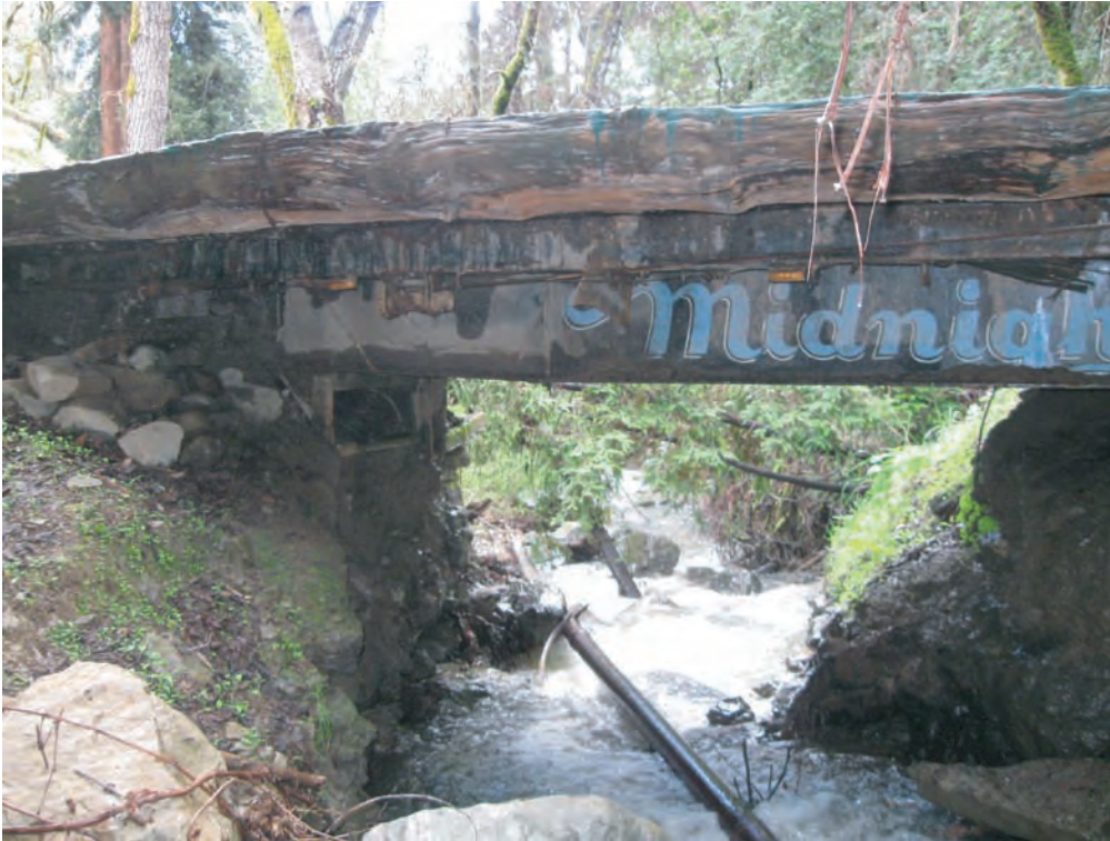
Photograph 1. Existing Bridge at 900 Doolan Canyon Drive. Photograph by CGS, March 3, 2010
