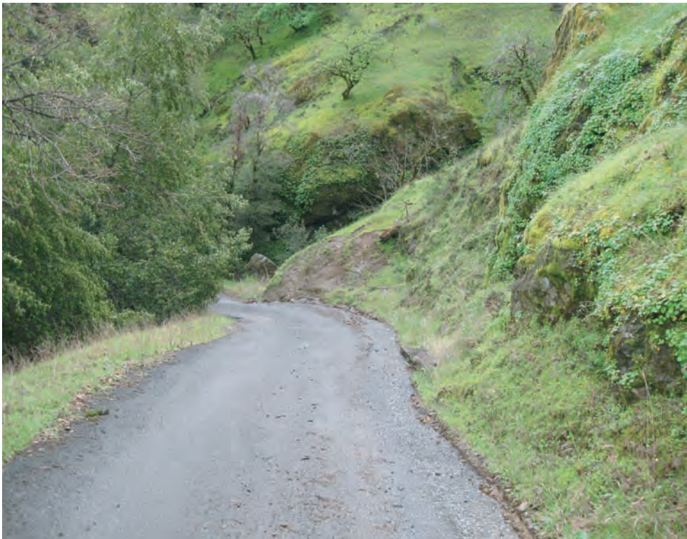
Photograph 2. Paved road ascending from bridge. Photograph by CGS, March 3, 2010.
