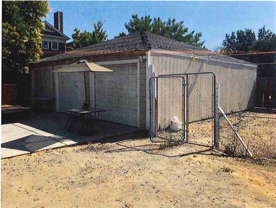
9. View of northeast corner of garage
