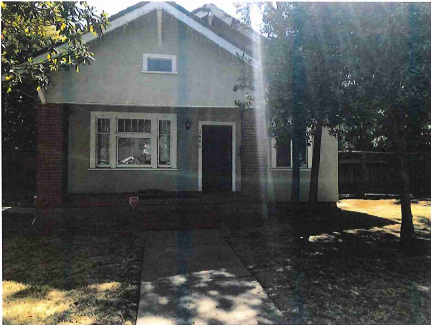
2. View of northeast side residence from Lincoln Ave., facing southwest
