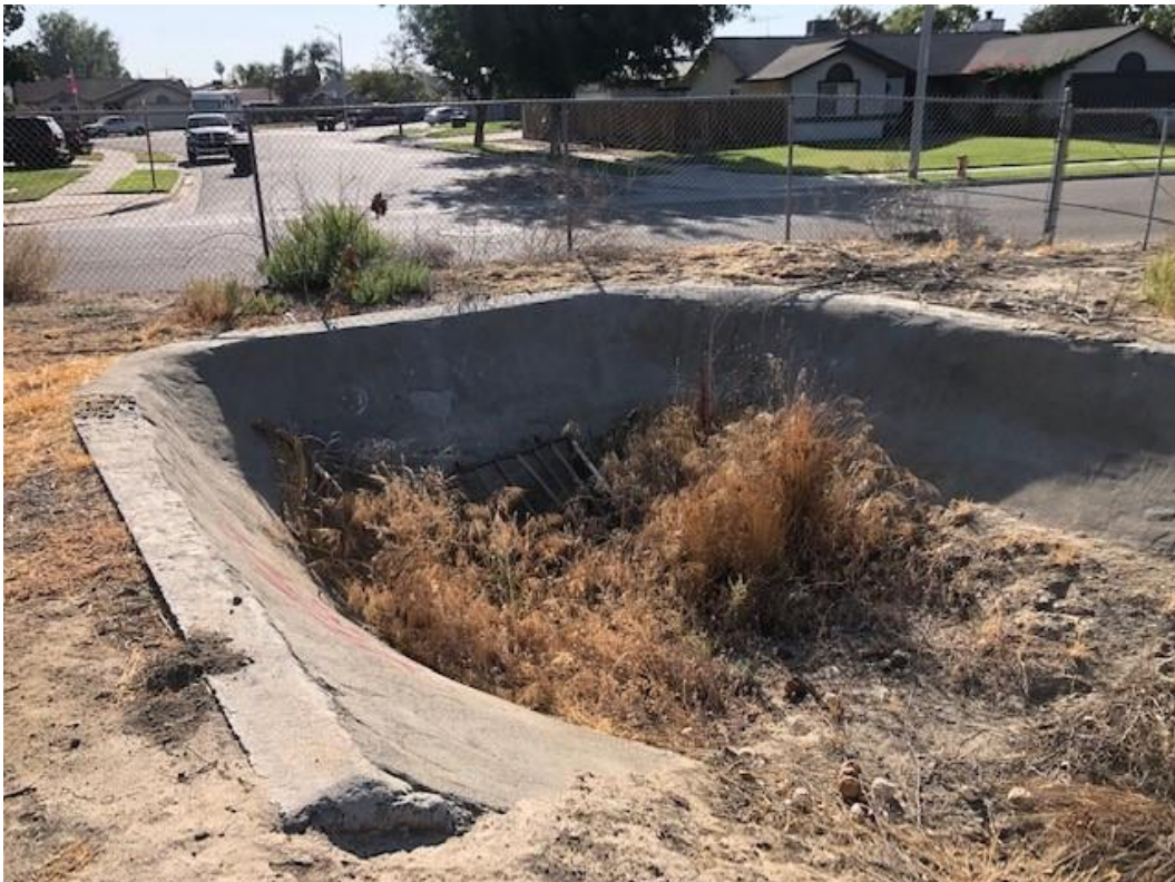
B) View looking east of the irrigation feature at the eastern edge of the project area. 8-18-2022. Acc. #2022IMG8378
