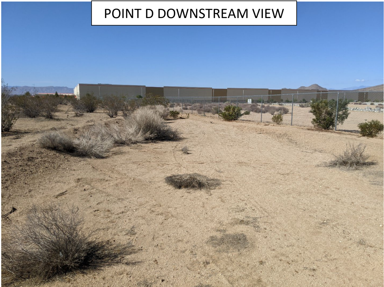
FIGURE 5, cont: PHOTOGRAPHS OF SITE
