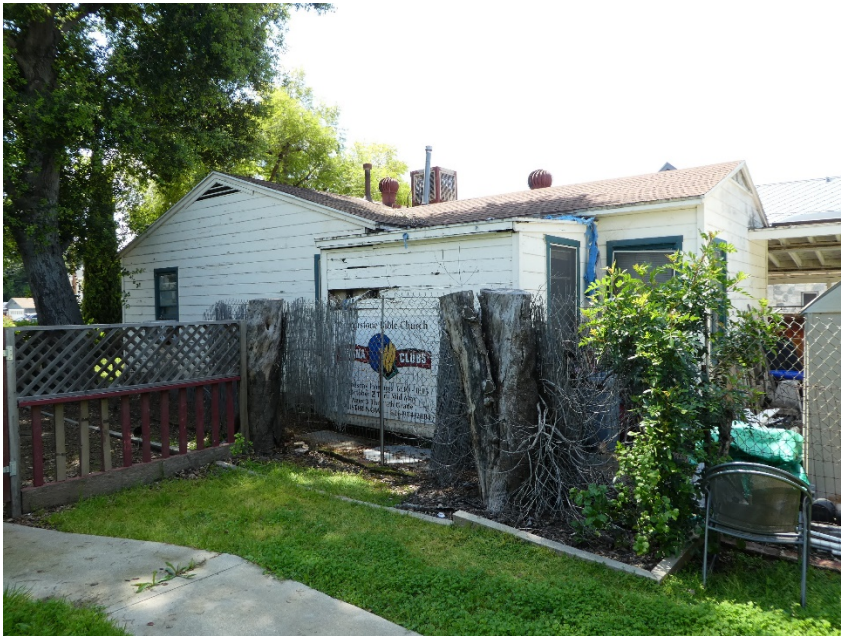
117 E. Whitcomb Avenue. View of the east façade, looking southwest.
