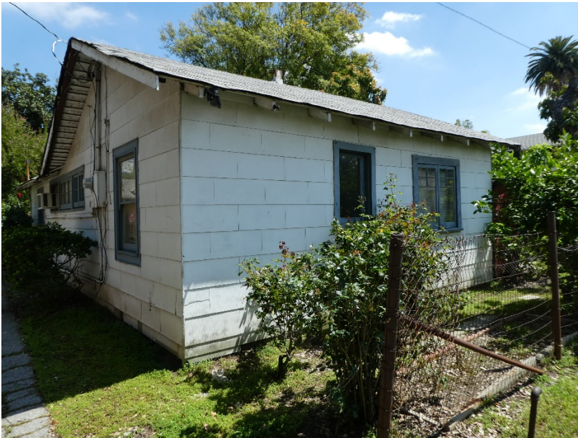
415 N. Vista Bonita Avenue. View of west façade, looking west southeast.
