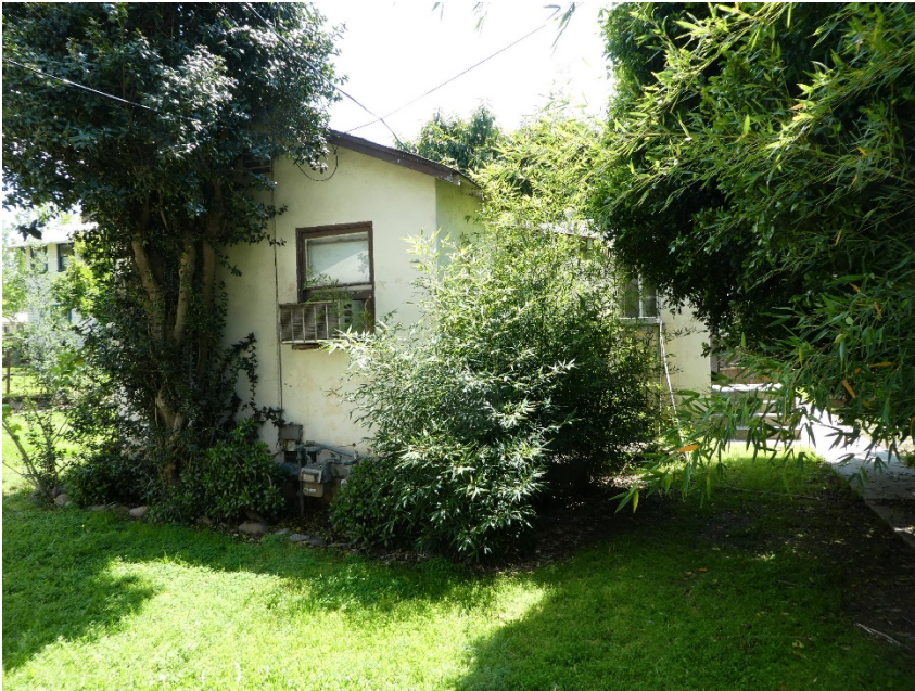
127 E. Whitcomb Avenue. View of north façade, looking south.
