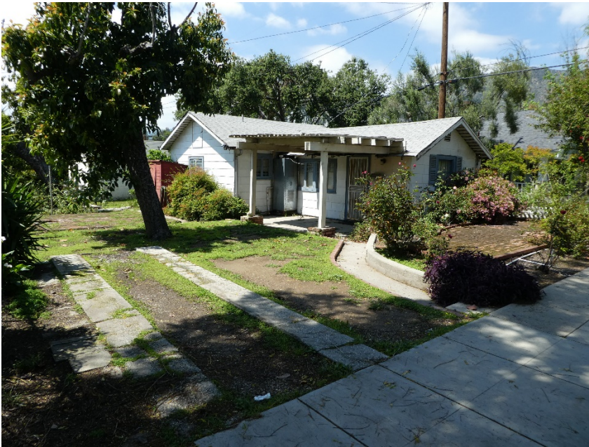
415 N. Vista Bonita Avenue. View of south and east facades, looking northwest.
