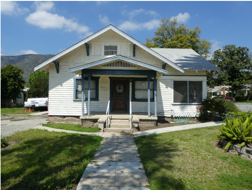
131 E. Whitcomb Avenue. View of south (primary) facade, looking north.
