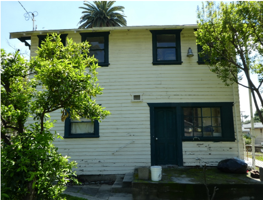
131 E. Whitcomb Avenue. View of north façade, looking south.
