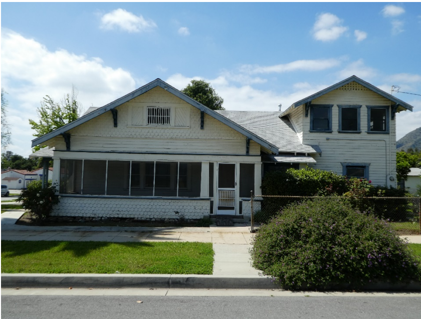
131 E. Whitcomb Avenue. View of east façade with screened porch, looking west.
