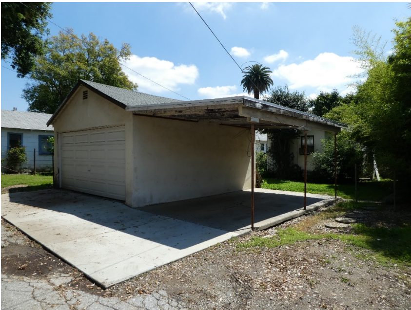
127 E. Whitcomb Avenue. View of garage with carport, looking southeast.
