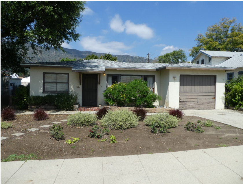
125 E. Whitcomb Avenue. View of the south (primary) façade, looking north.
