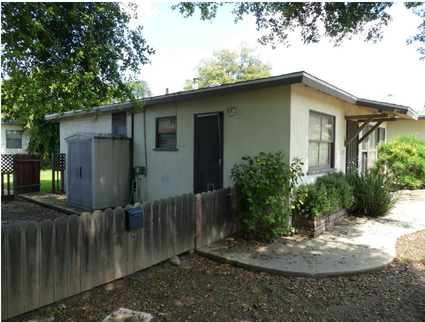
125 E. Whitcomb Avenue. View of the west façade, looking northeast.
